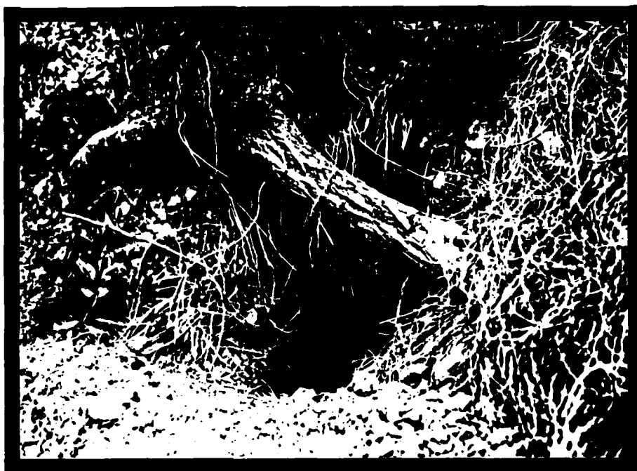
Photo 5 Animal Burrow on downstream slope near center of dam.
