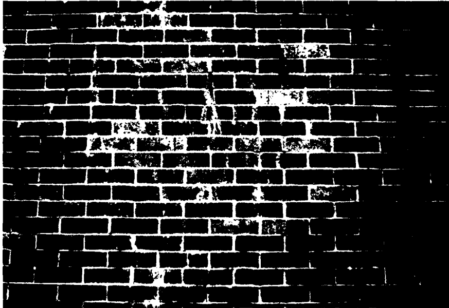
Figure 2. Typical efflorescence on exterior wall
