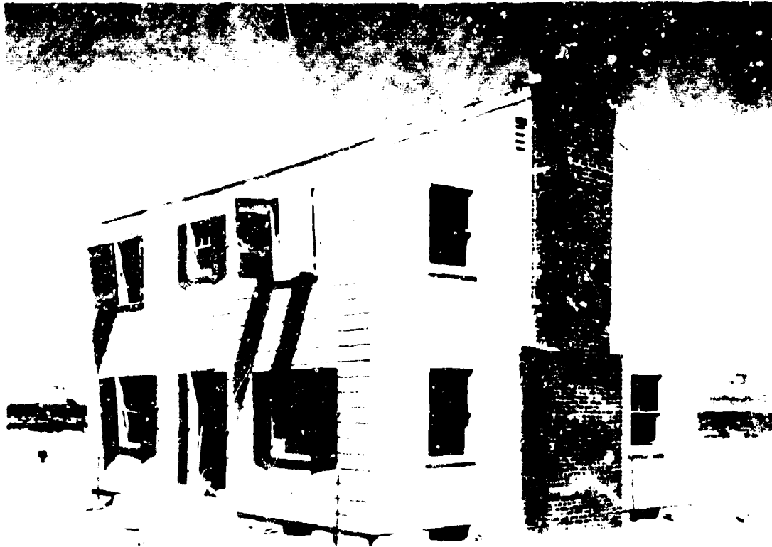
Figure 5.65. Strengthened wood-frame house after a nuclear explosion (2.6 psi peak overpressure).
