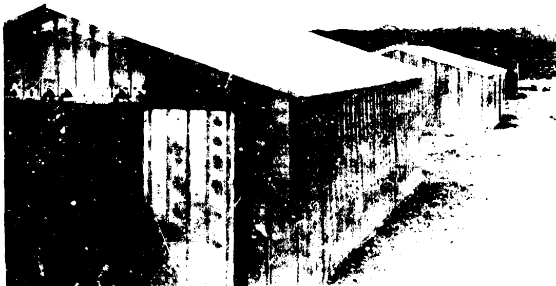
Figure 5.37a. Rigid steel-frame building before a nuclear explosion, Nevada Test Site.
