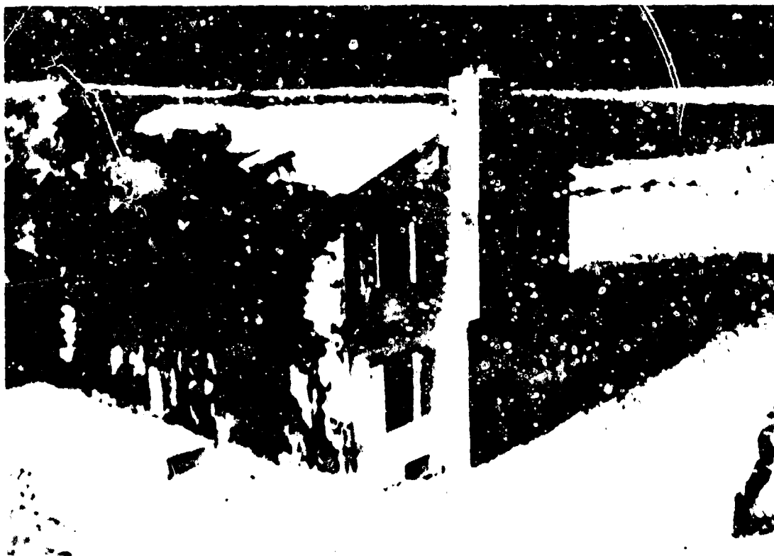
Figure 7.28a. Thermal effects on wood-frame house 1 second after explosion (about 25 cal/cm 2 ).
