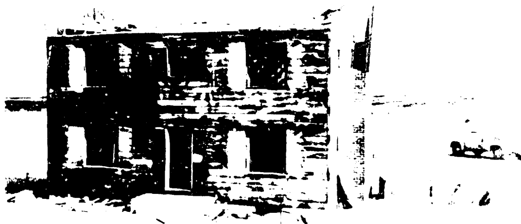
Figure 5.64. Strengthened wood-frame house after a nuclear explosion (4 psi peak overpressure).
