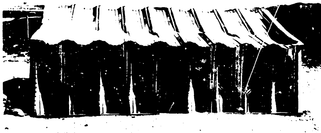
Figure 5.44. Self-framing corrugated steel panel building after a nuclear explosion (3.1 psi peak overpressure).
