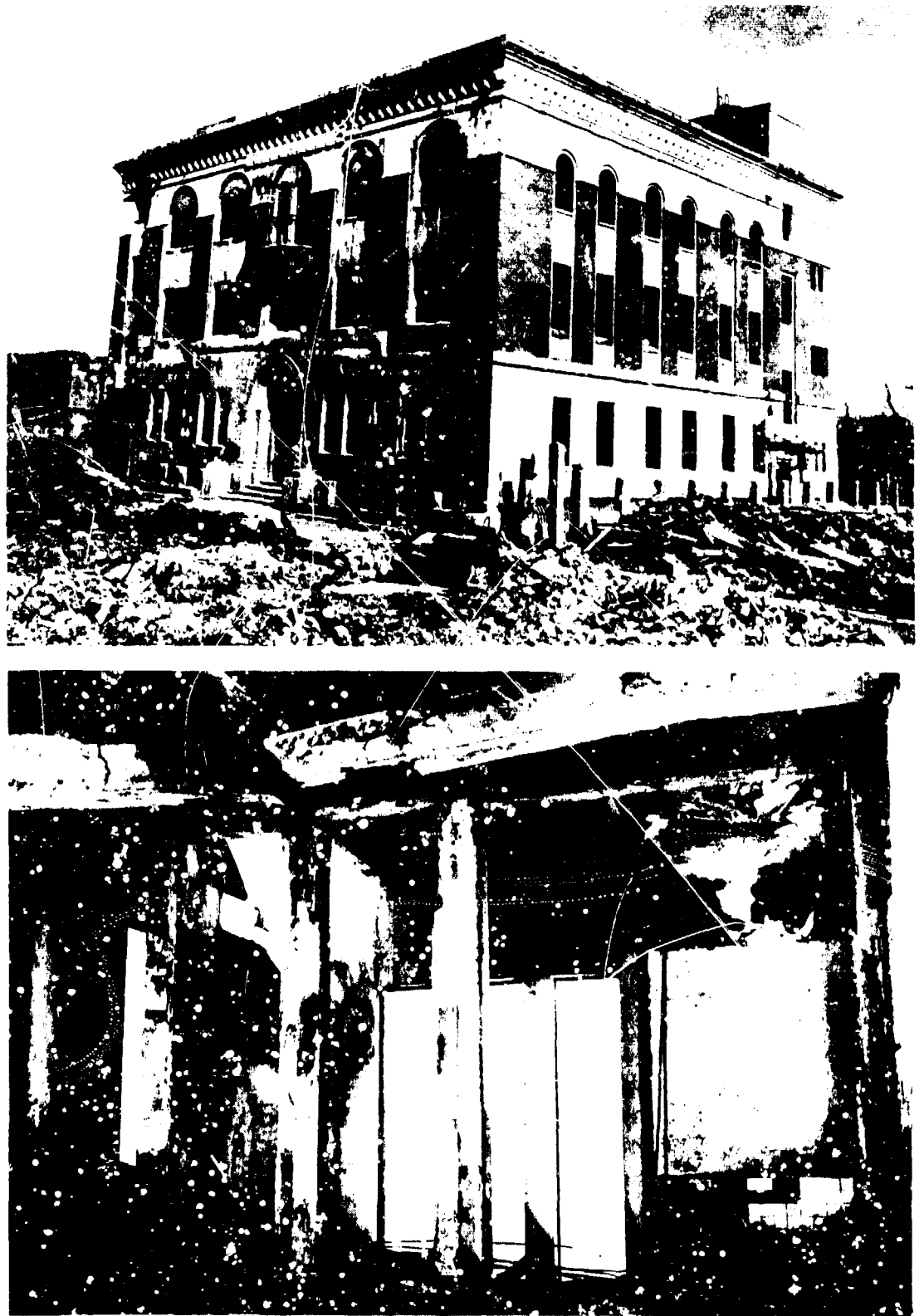
Figure 5.20a. Upper photo: Reinforced-concrete, aseismic structure; window fire shutters were blown in by blast and the interior gutted by fire (0.12 mile from ground zero at Hiroshima). Lower photo: Burned out interior of similar structure.
