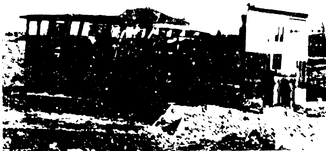
Figure 5.22b. Effects of horizontal loading on wall facing explosion (0.4 mile from ground zero at Nagasaki).
