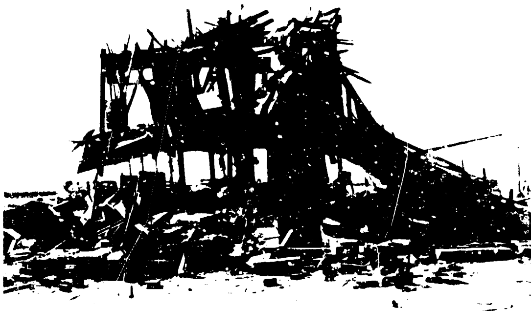
Figure 5.67. Unreinforced brick house after a nuclear explosion (5 psi peak overpressure).
