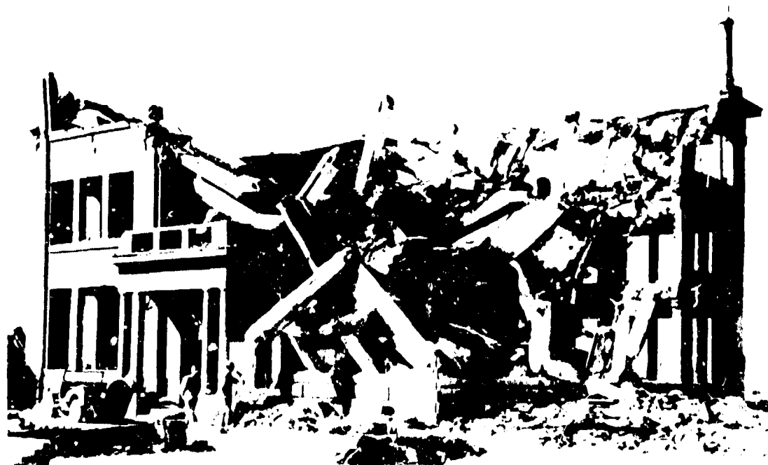
Figure 5.20b. Three-story, reinforced-concrete frame building: walls were 13-inch thick brick panel with large window openings (0.13 mile from ground zero at Hiroshima).
