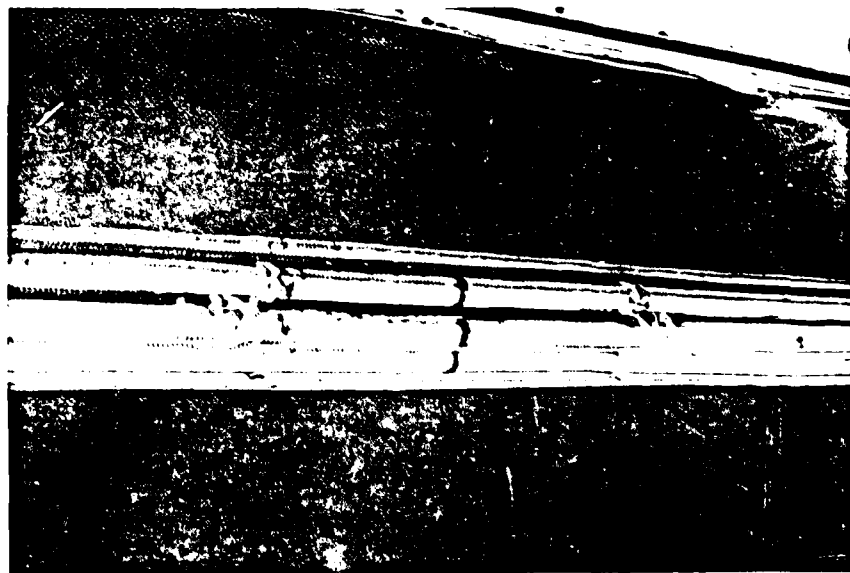
FIGURE 139. KING POST DIVIDER INSTALLED AND LACED INTO BRIDGE CABLE
