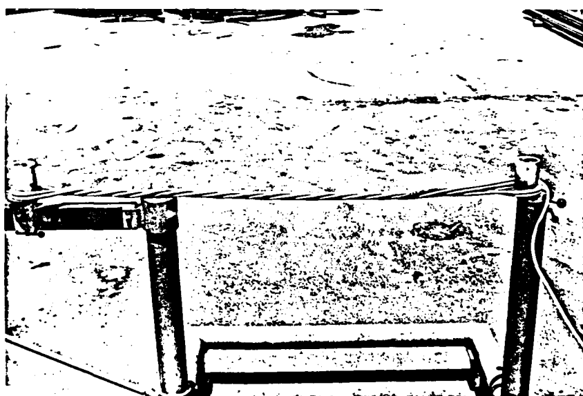
FIGURE 53. CONTINUATION OF PLAITING OF LEFT LAY STRANDS
