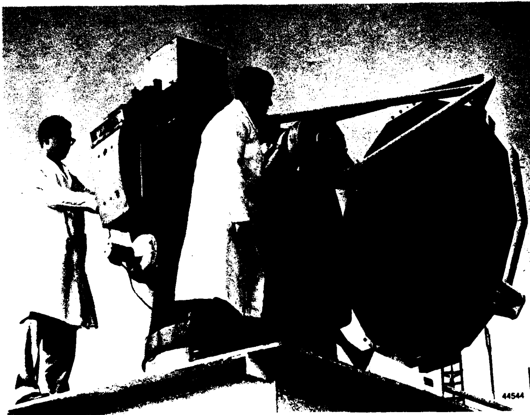
FIRST MONOPULSE RADAR
