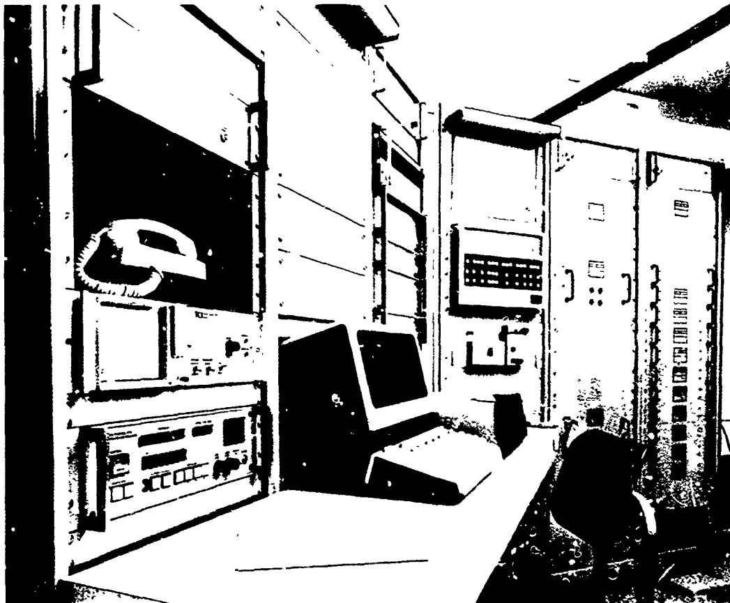
Fig. 2 Electronic Equipment at Typical DF Site
