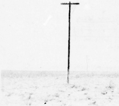
Pole line after explosion -- 1000 yds. Second pole is down from blast.
