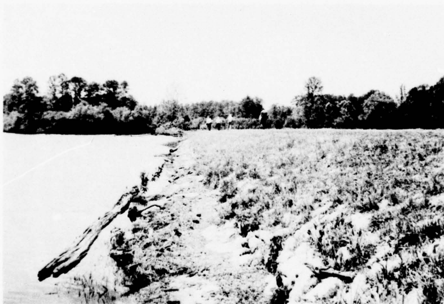
PHOTOGRAPH NO. 2 Upstream Face of Dam
