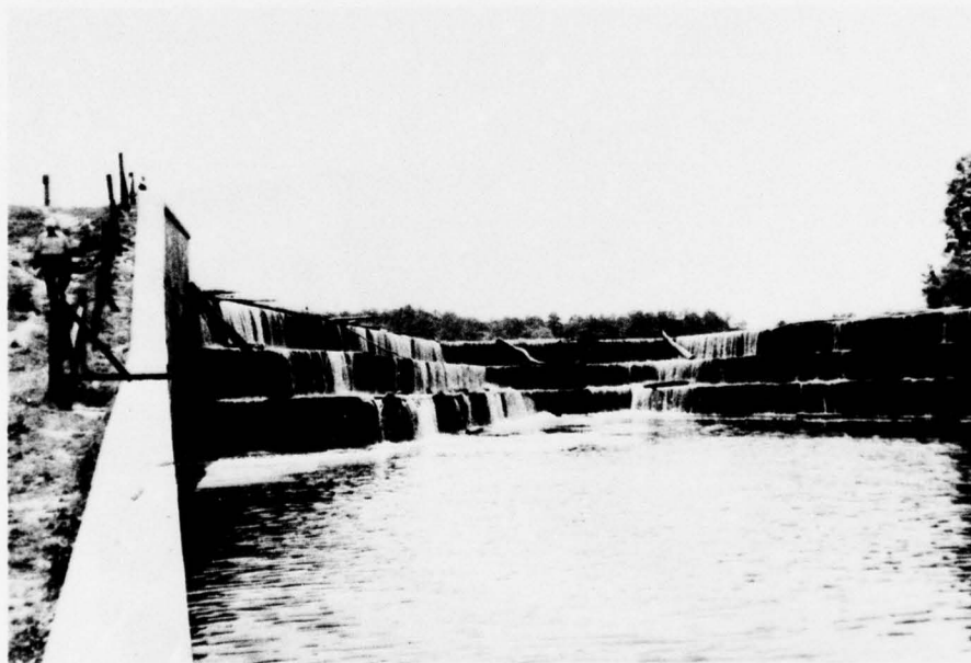
Spillway - Front View
