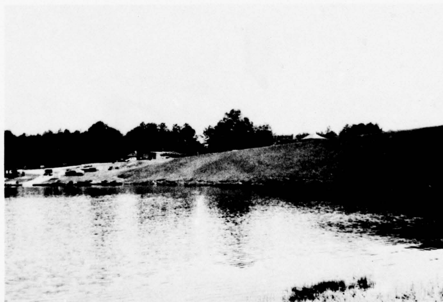
PHOTOGRAPH NO. 4 Face of Dam
