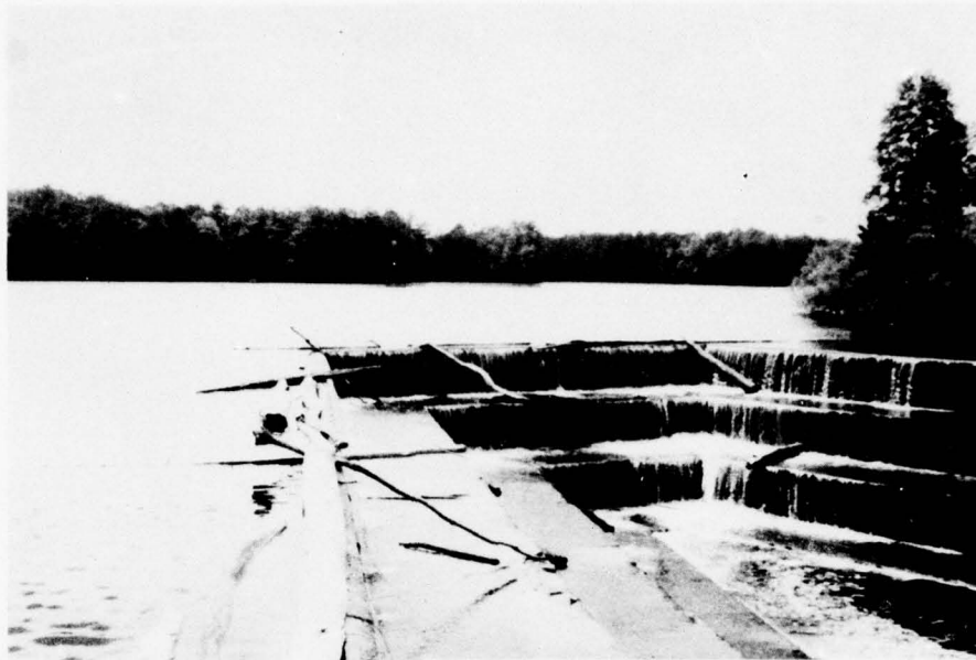
PHOTOGRAPH NO. 3 Spillway
