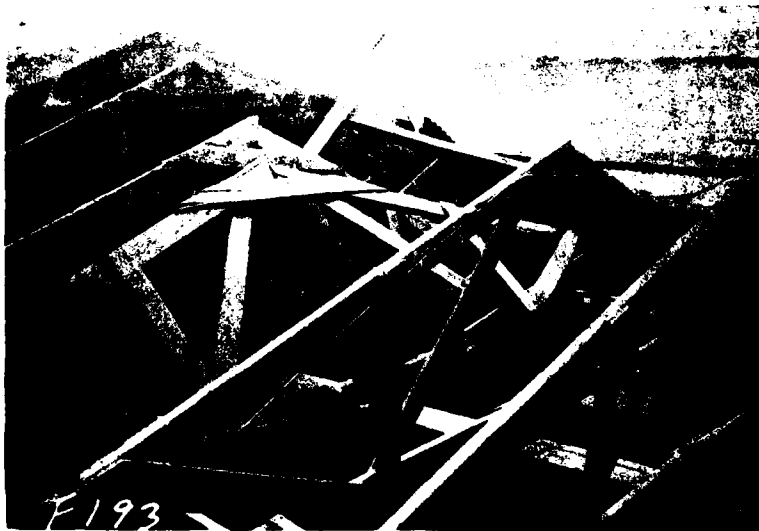
Fig. 4.20 Postshot, 3.5ab, Damaged Corrugated Steel Roof Panel (Note greater damage to trusses and purlins as compared to 3.5aa, Fig. 4.18)
