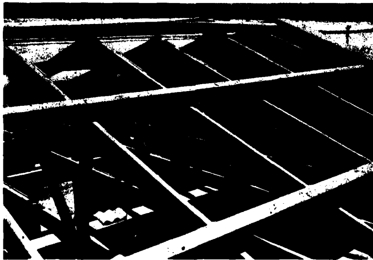
Fig. 4.18 Postshot, 3.5aa, Damaged Corrugated Asbestos Board Roof Panel (Note damage to top purlin and to top chord of trusses)
