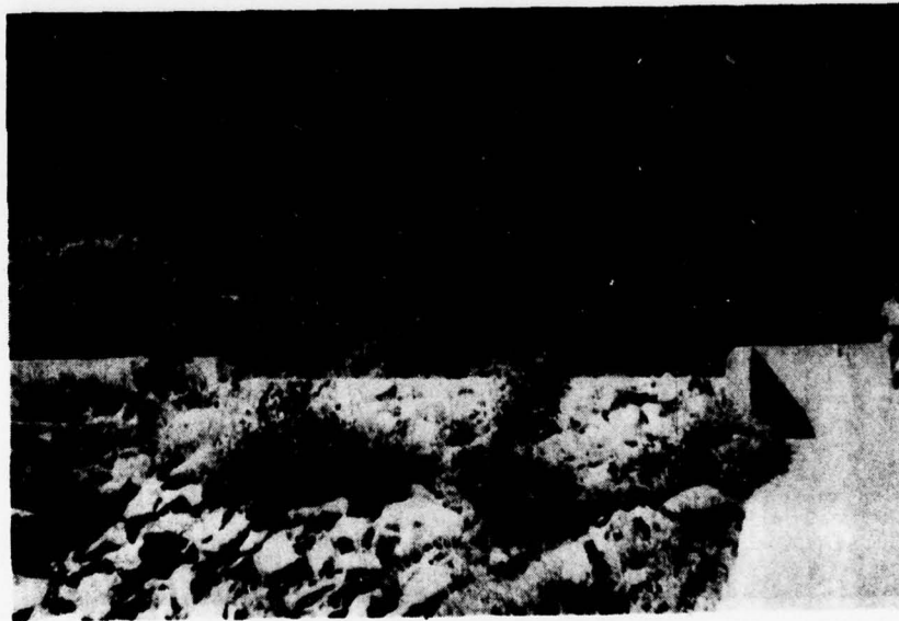
8. Lower diversion box culvert overflow weir. Reservoir is immediately below riprap area. See photo 16 for view of outlet in spillway area.
