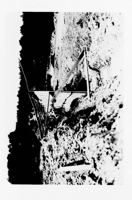
1929 CONSTRUCTION PHOTOGRAPH SHOWING WOODEN CUTOFF WALL AND BACKFILL TECHNIQUE.
