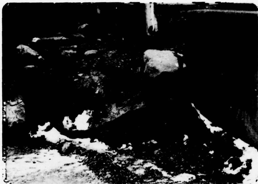
Erosion at left spillway/embankment junction.
