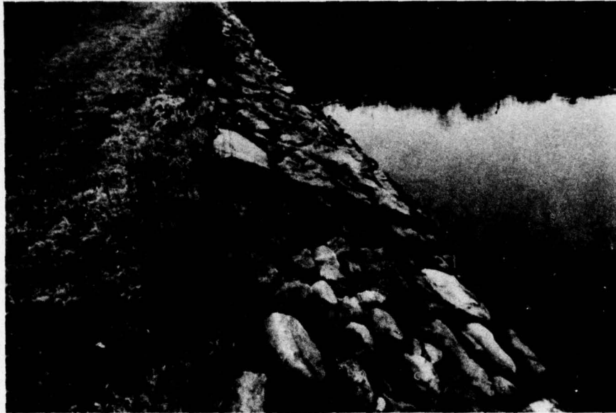
Photo 1 - Rock riprap extends to the crest of the embankment. (12-2-78)
