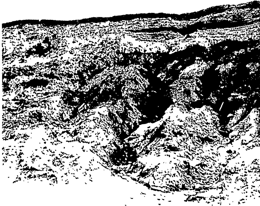
Figure 1-G12. Erosion of bluff at Highland Light Coast Guard Station
