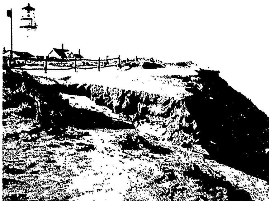
Figure 1-G11. Highland Light Coast Guard Station showing gulley caused by surface runoff
