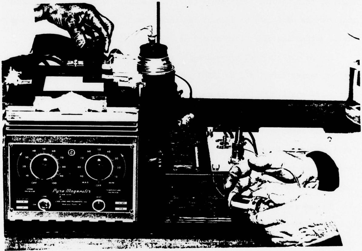
FIGURE 1 - Radiometric measurement of initial temperature of specimen and skin site.
