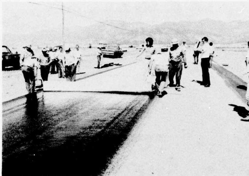
Photo 47. Fort Carson--placement of Mirafi 140 fabric
