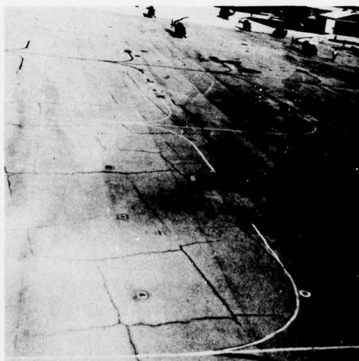
Photo 78. Fort Stewart--general view of condition of apron pavement prior to overlay
