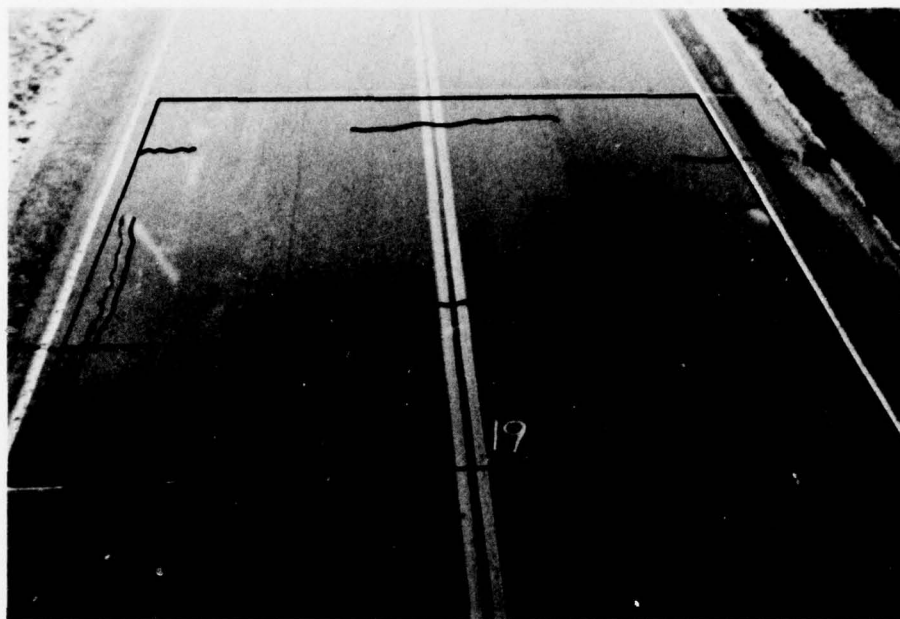
a. Condition of surface prior to overlay
