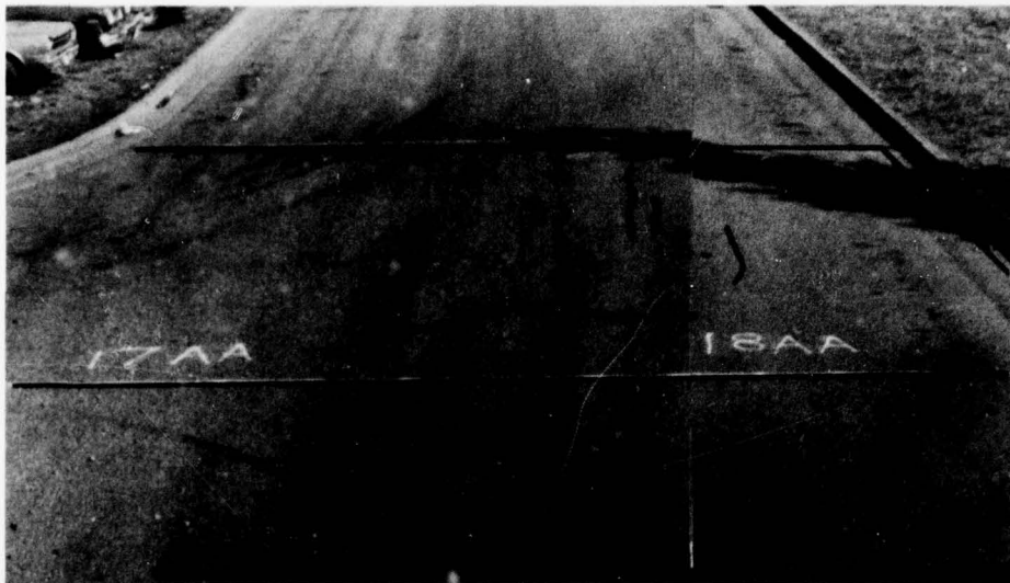
a. Condition of surface prior to overlay
