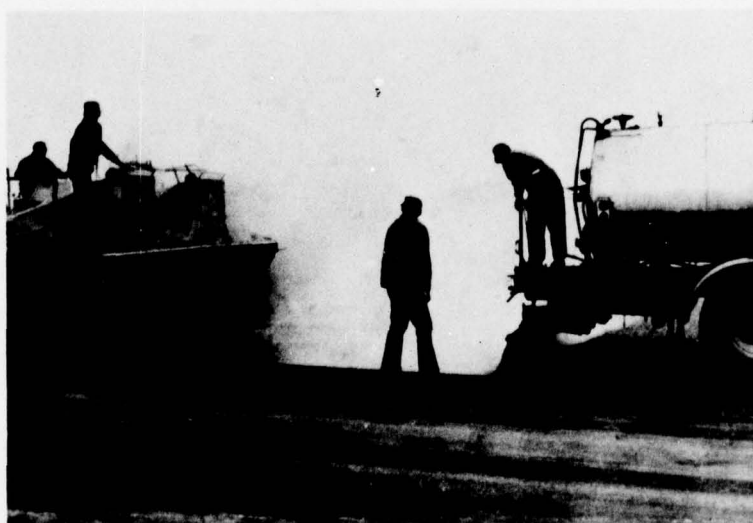
Photo 16. Fort Devens--considerable smoke from hot asphalt rubber
