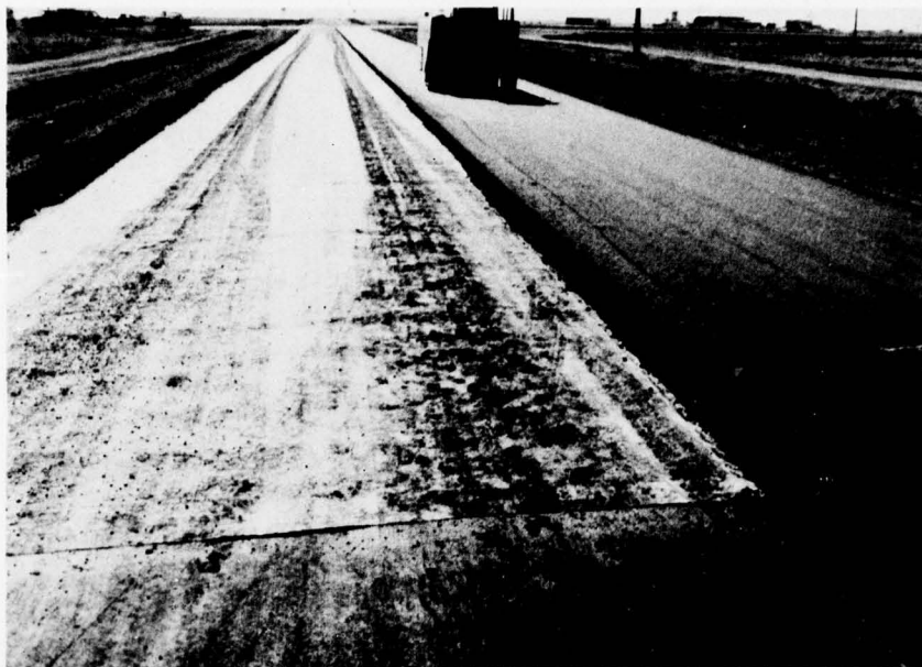
Photo 57. Fort Carson--overlay 1-1/2 in. thick placed over a fabric section
