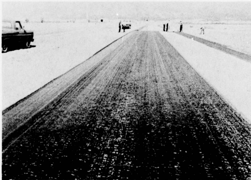
Photo 44. Fort Carson--application of tack very light, about 0.15 gal/sq yd
