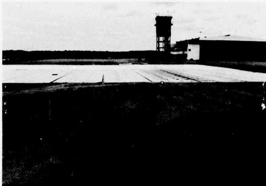
Photo 13. Fort Devens--fabric test sections on apron; Bidim C-22 placed in direction of paving; Mirafi 140 transverse to paving
