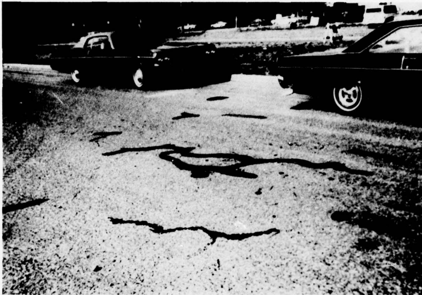
Photo 33. Fort Lewis--cracks on Faith Avenue sealed with AR-4000 asphalt
