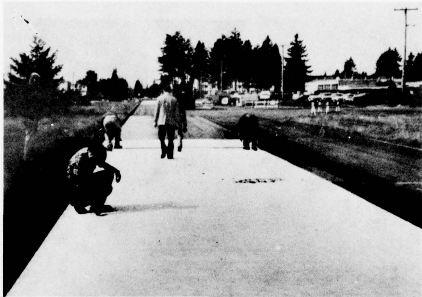
Photo 39. Fort Lewis--placement of Mirafi 140 fabric
