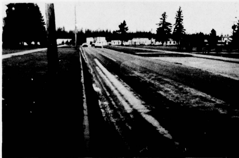
Photo 58. Fort Lewis--asphalt-rubber chip seal placed by Sahuaro ravelling in traffic wheel paths; note buildup of loose chips at curb line
