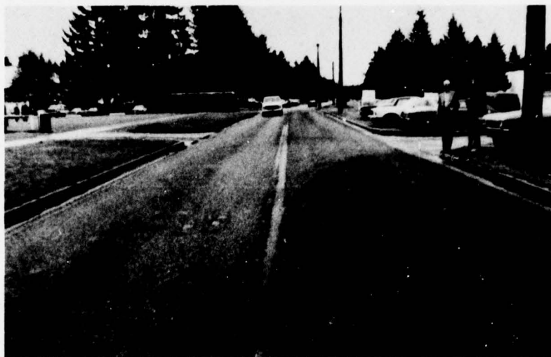
Photo 59. Fort Lewis--U. S. Rubber chip seal with bare spot at center line; area did not receive rubberized material during construction
