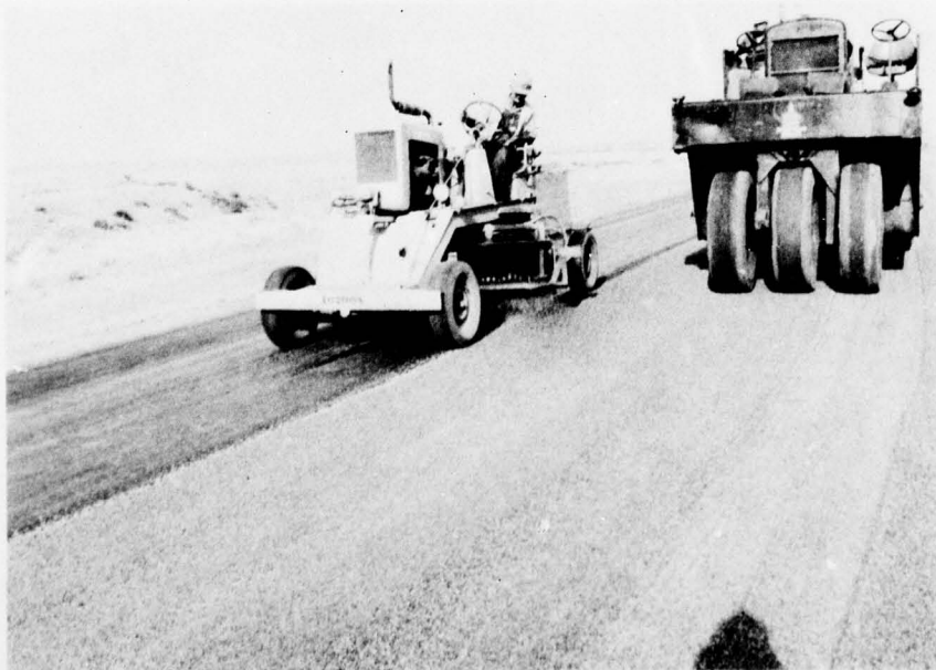
Photo 56. Fort Carson--brooming of edge joint and rolling cover aggregate
