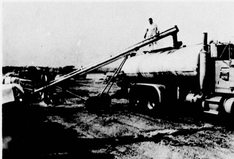
Photo 14. Fort Devens--addition of rubber to distributor for application on U. S. Rubber test section on NW-SE runway
