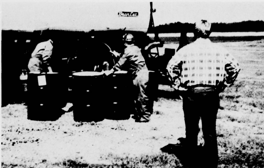
Photo 27. Fort Stewart--pumping kerosene into Sahuaro distributor
