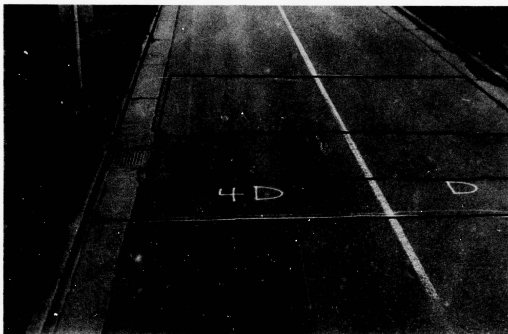
a. Condition of surface prior to overlay
