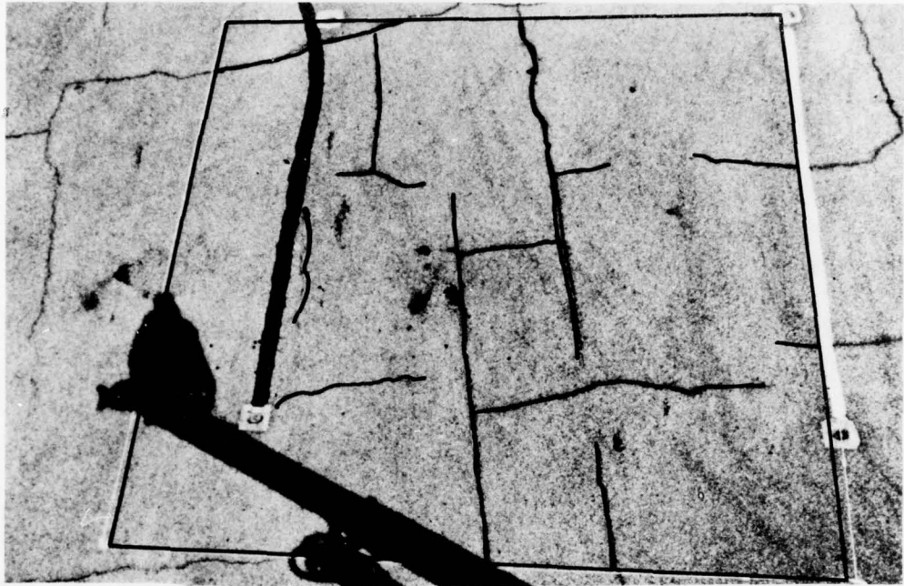
a. Condition of surface prior to overlay
