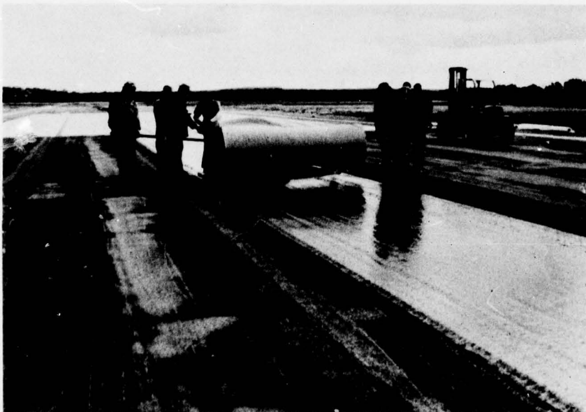
Photo 4. Fort Devens--placement of Bidim C-22 fabric on NW-SE runway; very difficult to place wrinkle free
