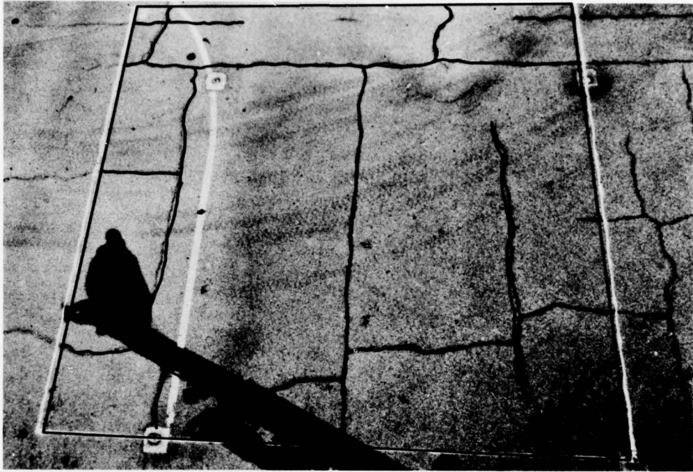
a. Condition of surface prior to overlay
