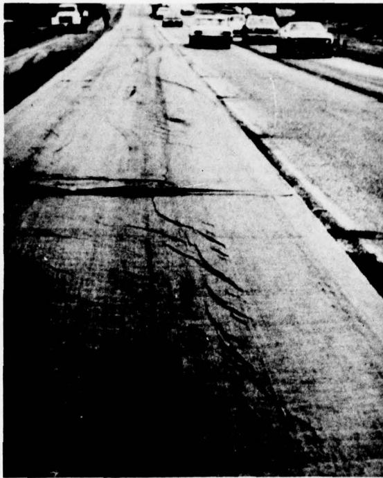
Photo 43. Fort Polk--Petromat fabric placed with considerable amount of wrinkles
