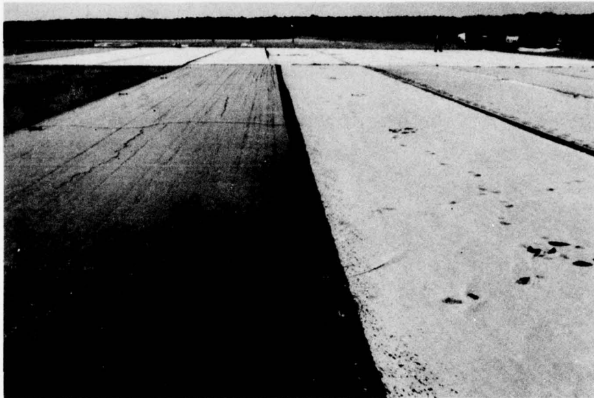
Photo 21. Fort Stewart--overlap of about 9 in. at joint; note no wrinkling of Bidim C-22 fabric
