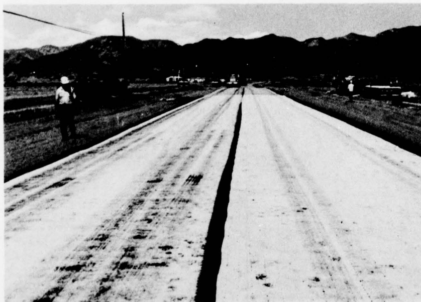
Photo 52. Fort Carson--tack material evident on surface of fabric
