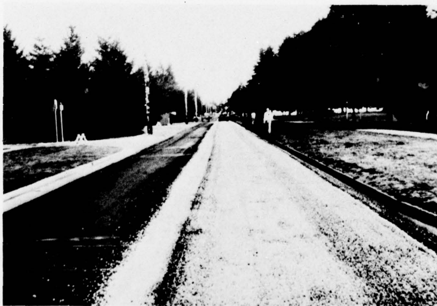
Photo 32. Fort Lewis--one lane of asphalt rubber and chips on Second Division Drive; joint has not been swept as yet for next lane
