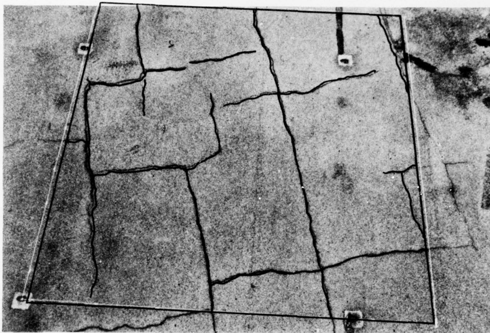
a. Condition of surface prior to overlay
