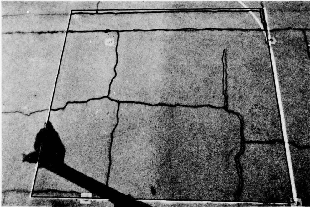
a. Condition of surface prior to overlay
