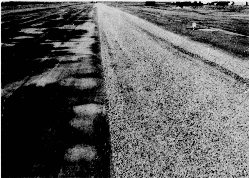
Photo 18. Fort Devens--asphalt rubber and chips after rolling
