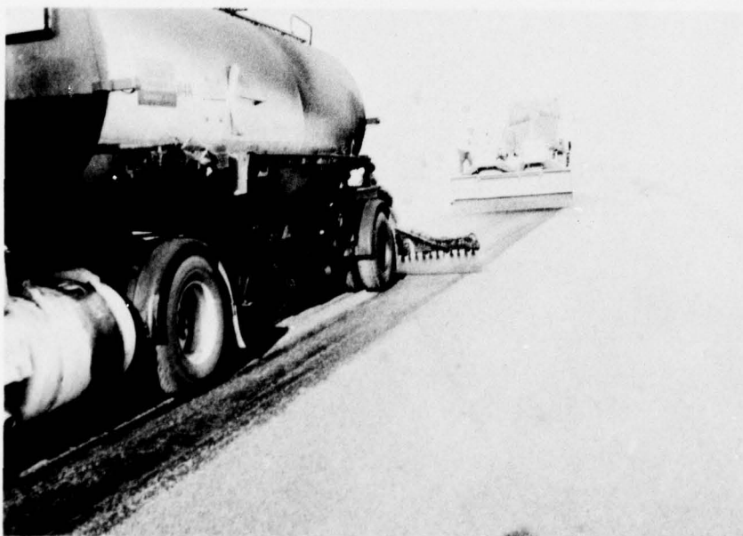
Photo 54. Fort Carson--application of asphalt rubber by Sahuaro distributor
