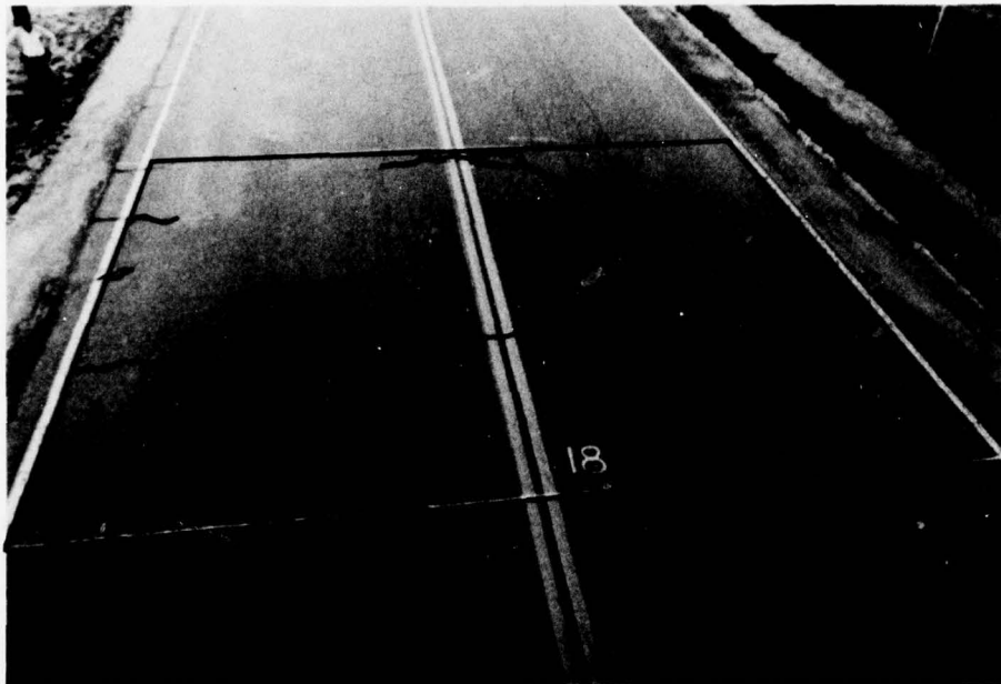
a. Condition of surface prior to overlay
