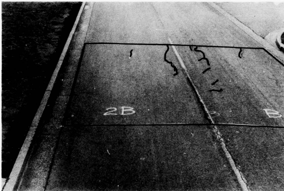
a. Condition of surface prior to overlay
