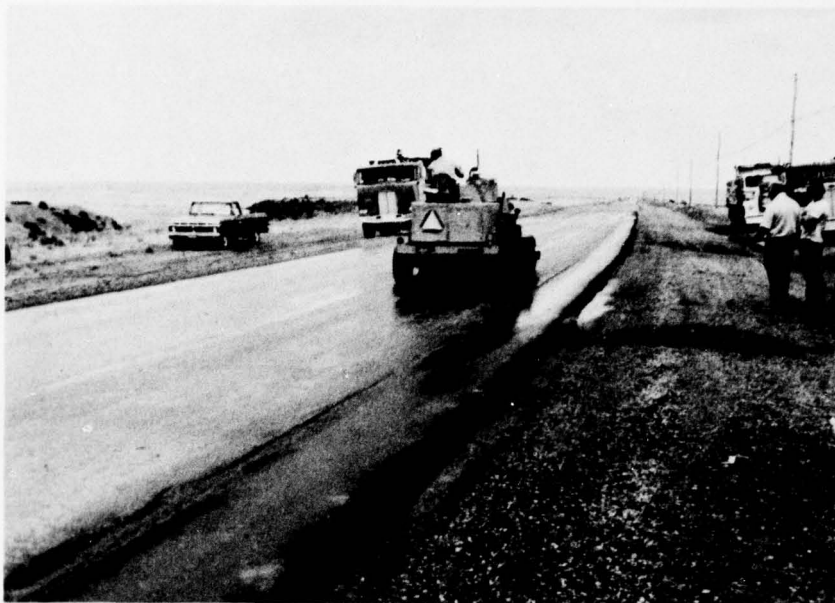
Photo 53. Fort Carson--brooming surface water from pavement in Sahuaro test area
