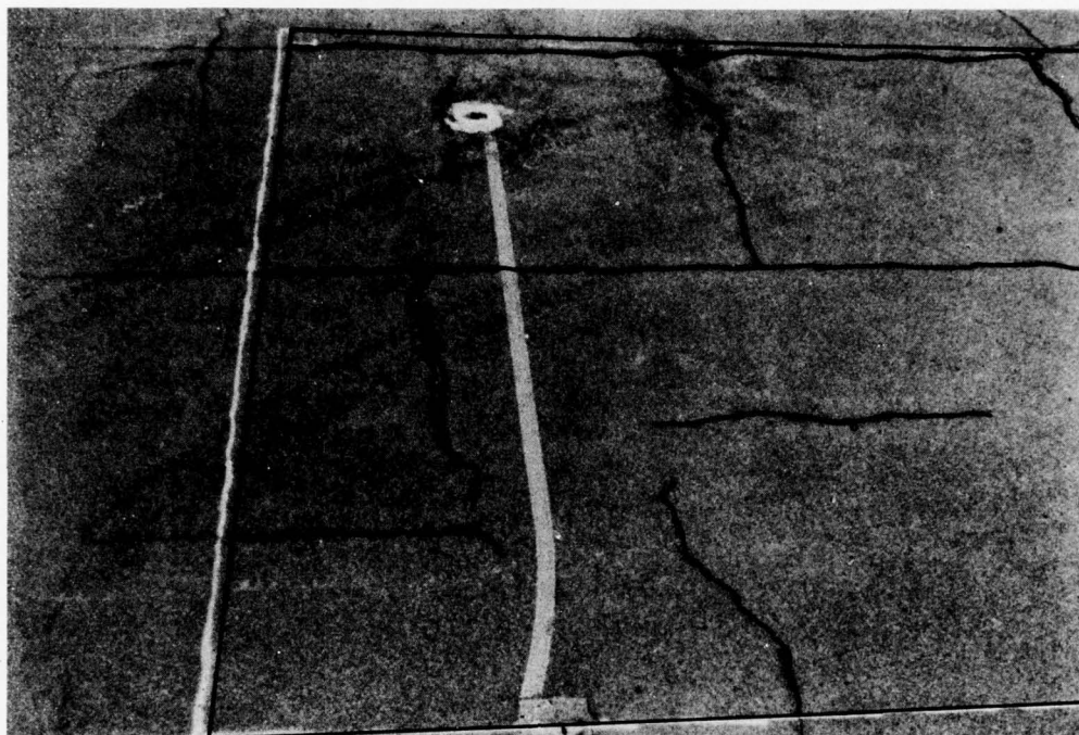
a. Condition of surface prior to overlay
