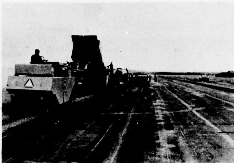
Photo 15. Fort Devens--aggregate spreader and rollers follow immediately behind distributor
