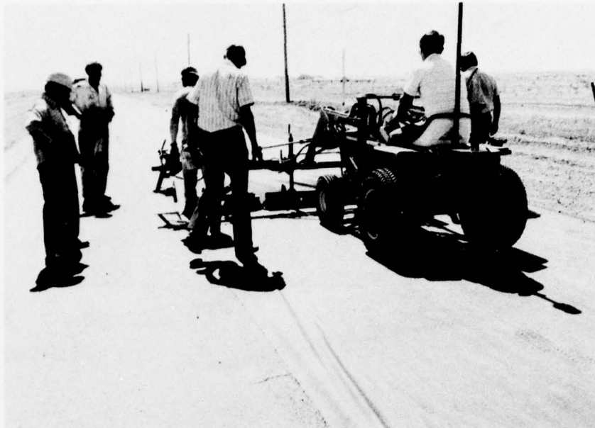
Photo 51. Fort Carson--Petromat fabric being placed relatively free of wrinkles
