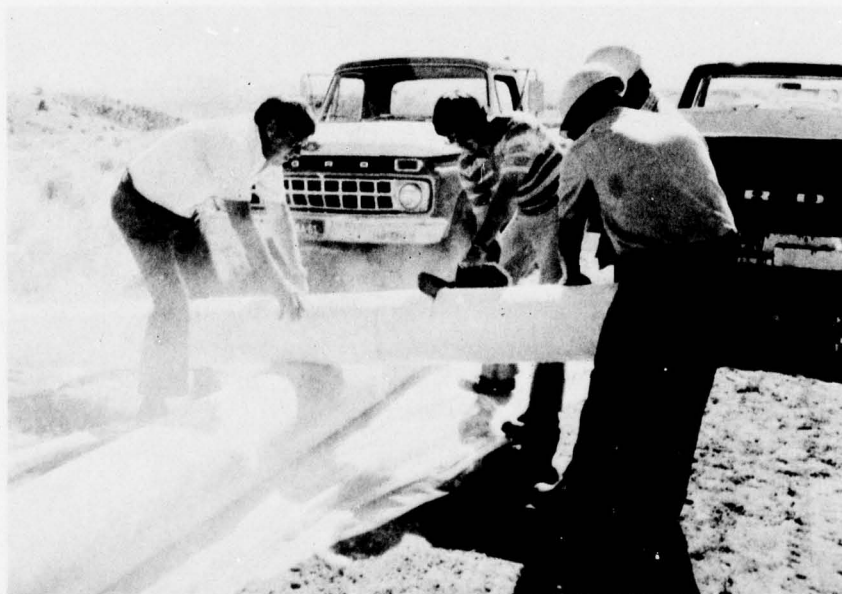
Photo 46. Fort Carson--Mirafi 140 fabric cut to 12-ft 6-in. width
