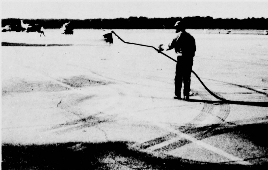
Photo 28. Fort Stewart--application of light tack coat over test area
