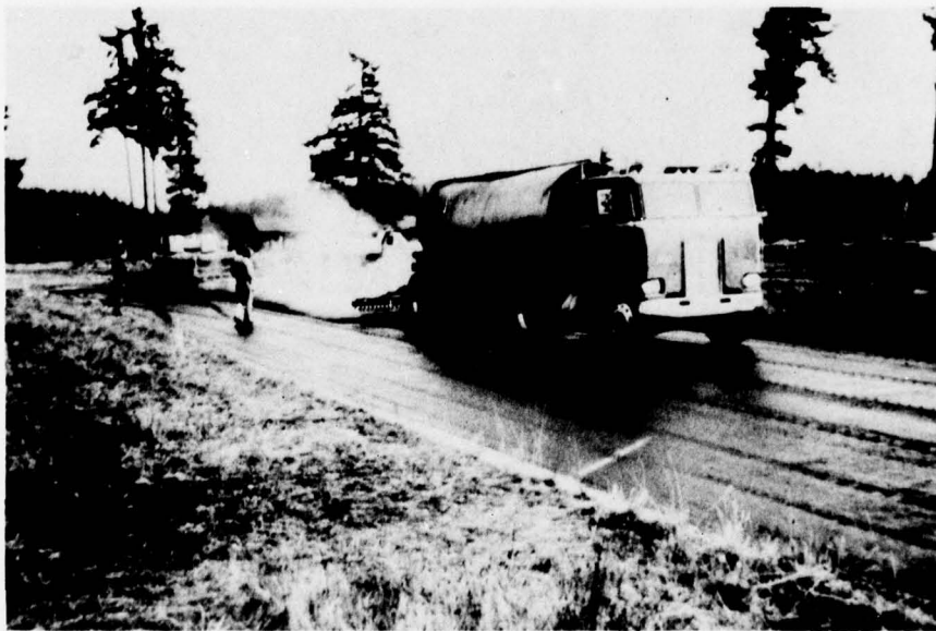
Photo 34. Fort Lewis--application of Sahuaro asphalt-rubber mixture on Faith Avenue
