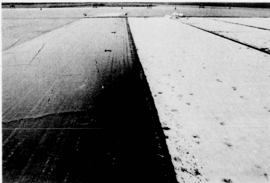
Photo 22. Fort Stewart--overlap of about 6 in.; note wrinkling of Mirafi 140 fabric
