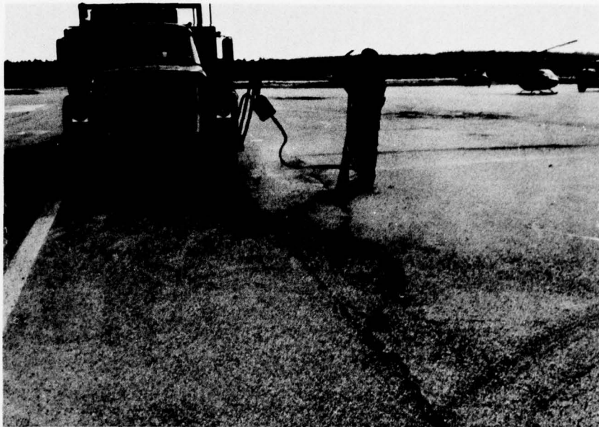
Photo 7. Fort Devens--cleaning of cracks on apron area prior to sealing
