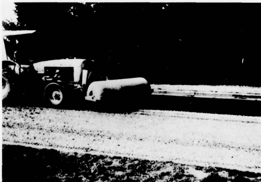
Photo 36. Fort Lewis--power broom used to sweep joints of loose aggregate
