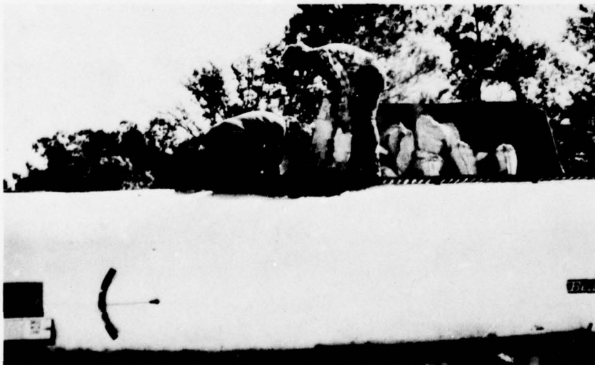
Photo 26. Fort Stewart--loading bags of rubber to Sahuaro distributor truck
