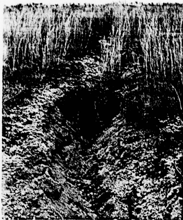
Erosion of downstream slope of dam
