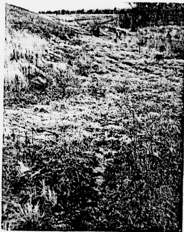
Seepage at downstream toe
