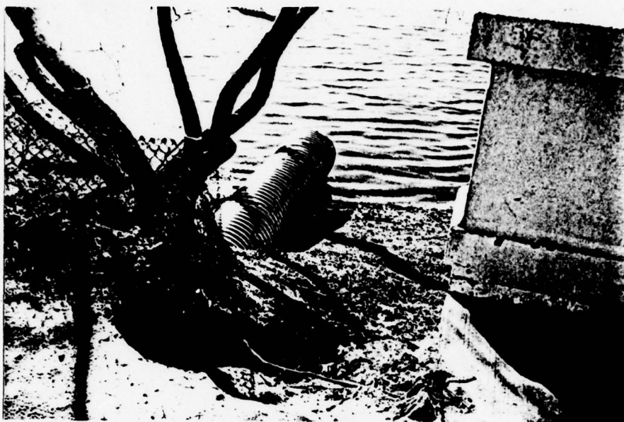
Roadway drain at S.E. wingwall
