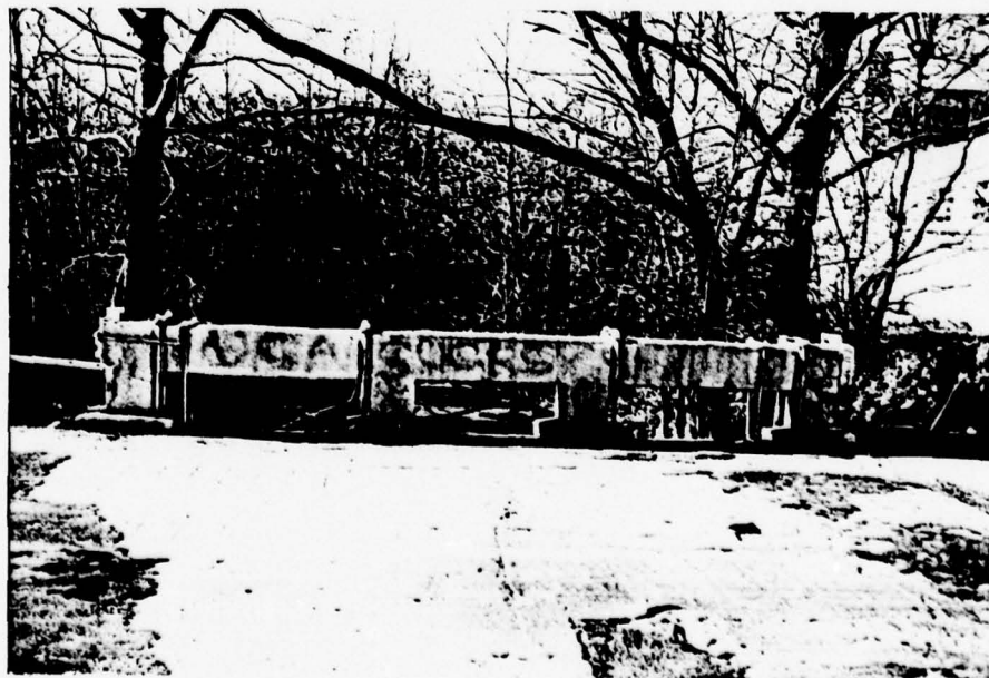
Bridge deck and rail
