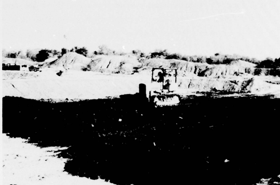
Figure B9. Spreading dredged material on plots
