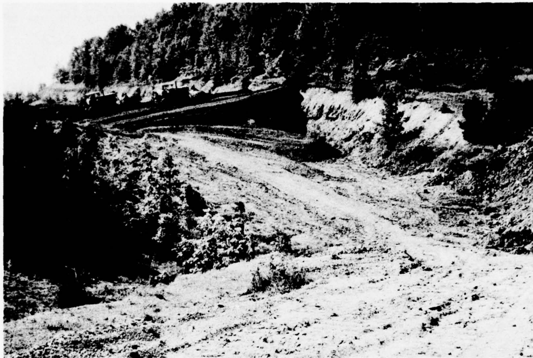
Figure 13. Backfilling of surface mined area (from McNay 35 )
