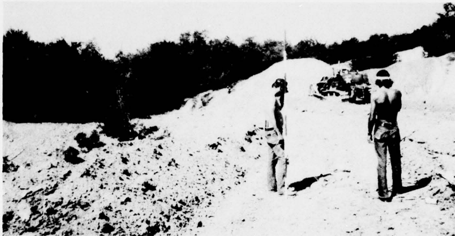
Figure B4. Leveling mine spoil ridges
