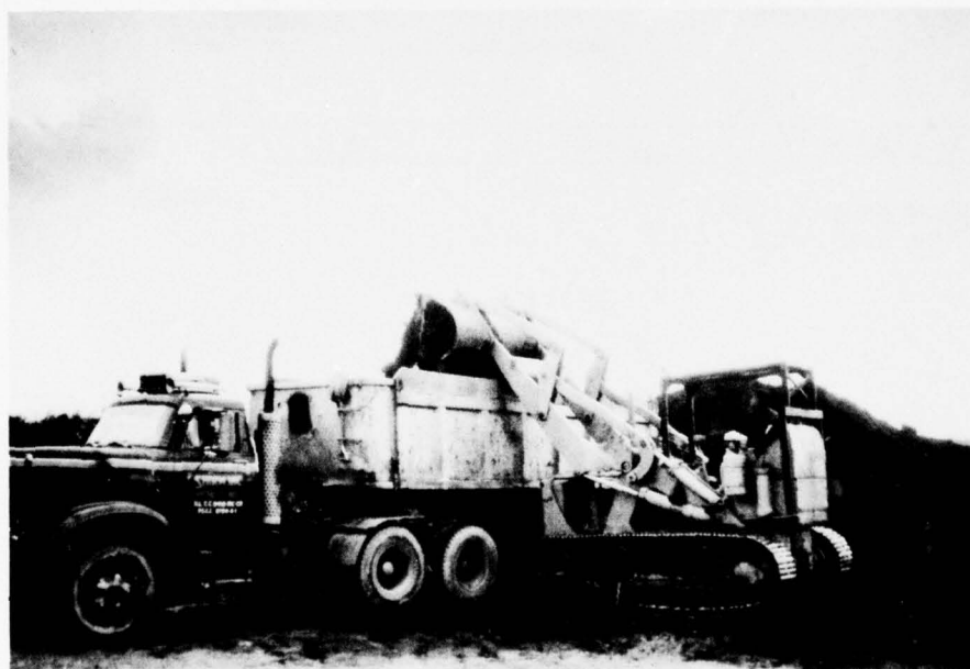
Figure B8. Loading dredged material at borrow area
