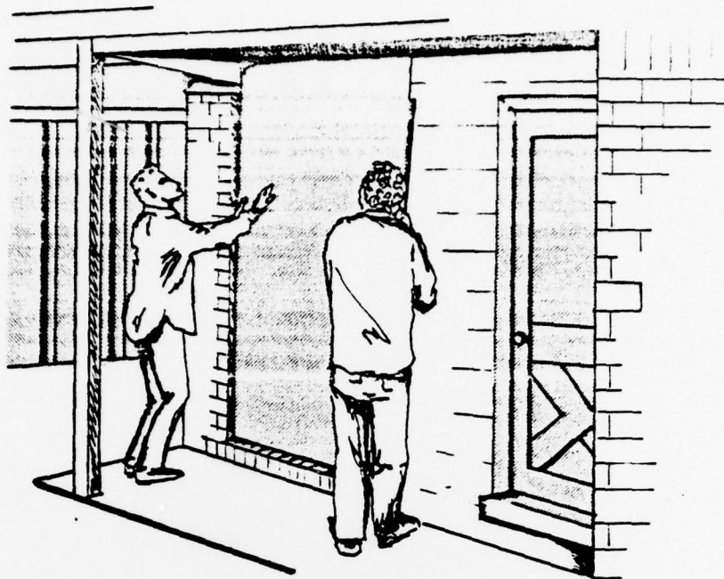
FIGURE A-2a. PLACING BOARDS OVER EXTERIOR WALL APERTURES.
