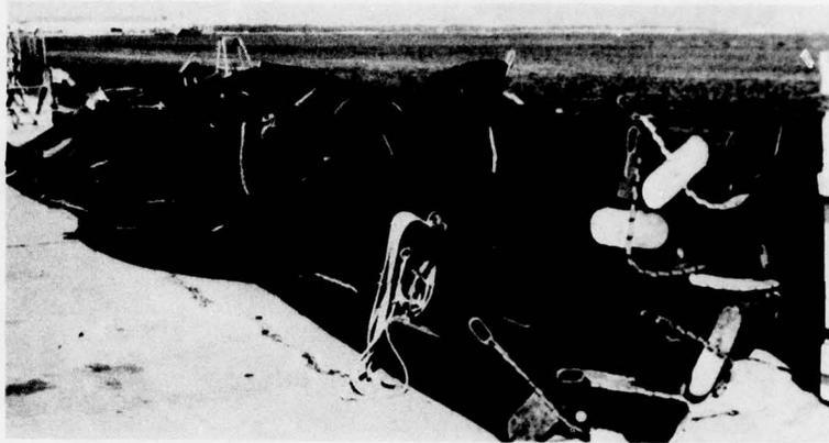
Figure 52. A spreader bar and lengths of Goodrich boom awaiting assembly.
