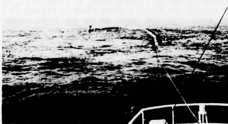
Figure 22. Crewmen in a Zodiac boat complete the Coast Guard boom mooring, while USCGC POINT LOBOS holds the position.
