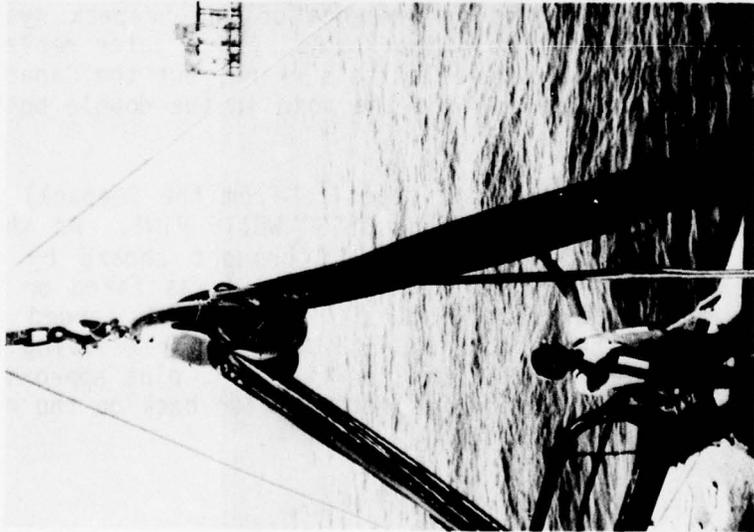
Figure 38. The Vikoma boom being retrieved through a Marco power block.
