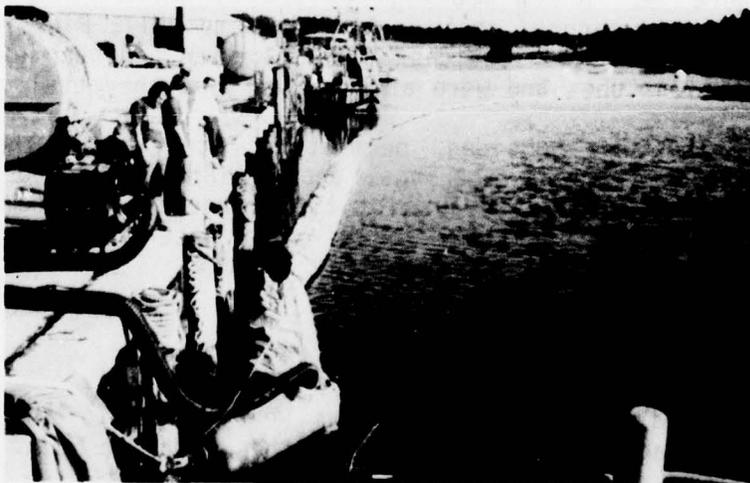
Figure 41. Inflating the Bennett boom at dockside.
