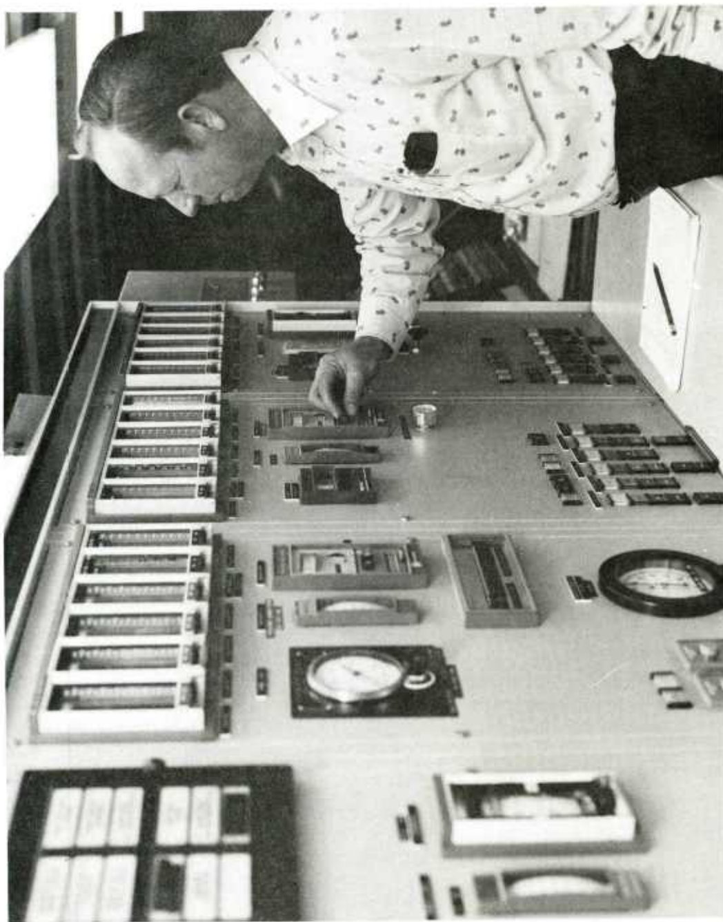
Figure 8. Incinerator instrumentation and control panel.
