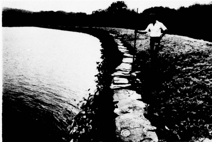
C. Riprap on Upstream Slope
