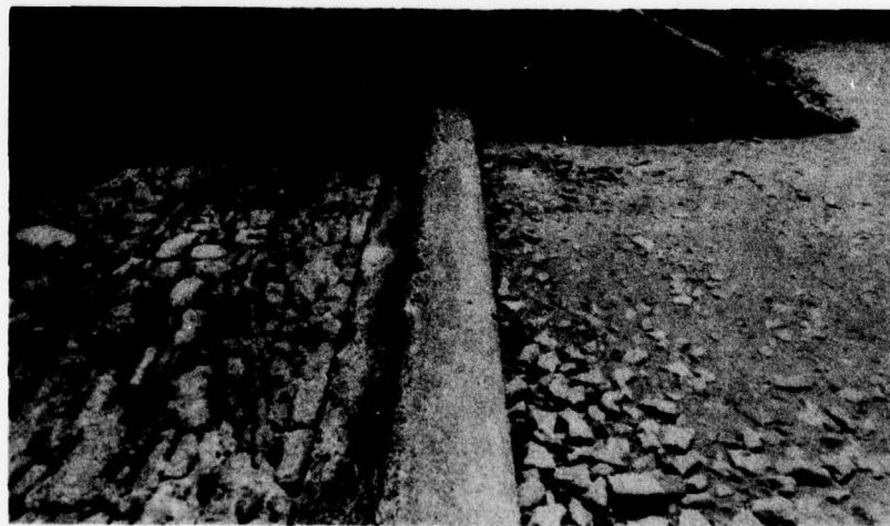
F. Concrete Spillway Weir and Masonry Apron.
