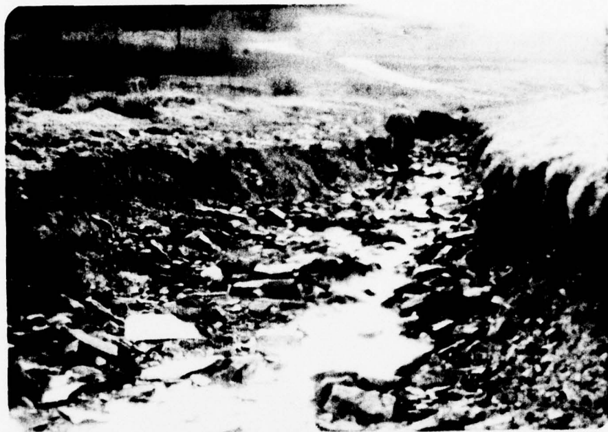
Photograph No. 7 Erosion in discharge channel.
