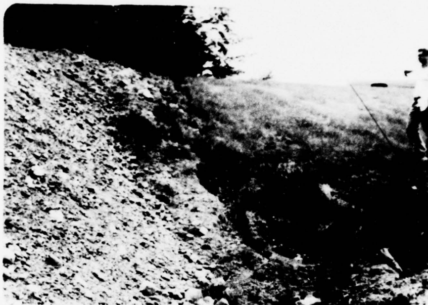
EROSION ON DOWNSTREAM EMBANKMENT SLOPE
