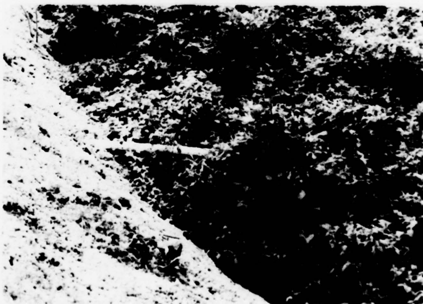
OUTLET PIPE FOR TOE DRAINAGE
