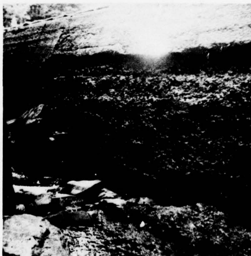
DOWNSTREAM FACE OF SPILLWAY SHOWING SPALLING AND UNDERMINING
