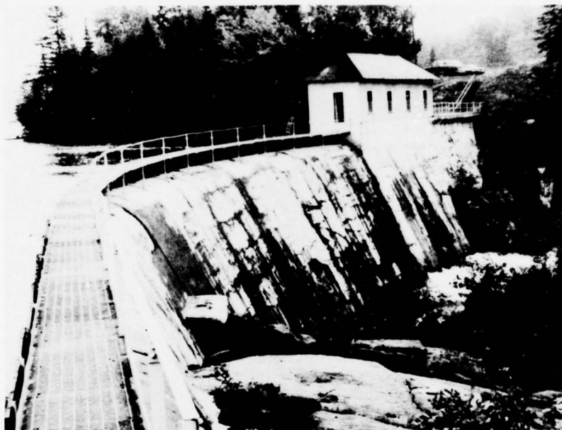
CONCRETE SPILLWAY AND GATE HOUSE
