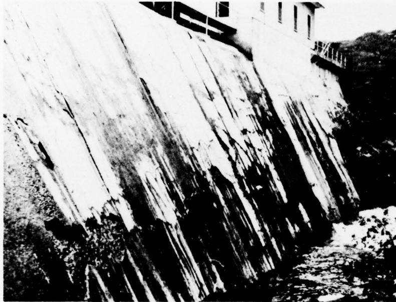
DOWNSTREAM SLOPE OF SPILLWAY
