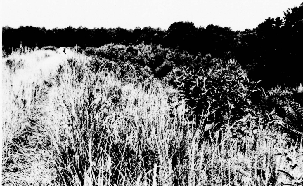
PHOTO 3. Brush and Trees Growing on Downstream Face Looking From Right Side
