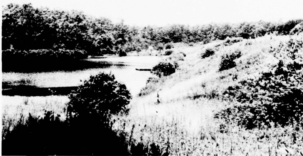
PHOTO 4. Brush and Trees on the Upstream Face Looking From Right Side
