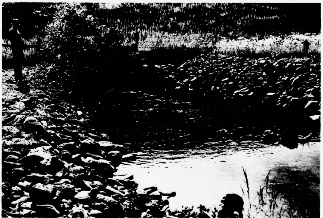
PHOTO 2. Stilling Basin at Downstream Outlet of Principal Spillway
