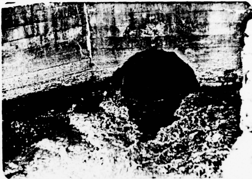
Photograph No. 7 "Blow-off" pipe discharging.
