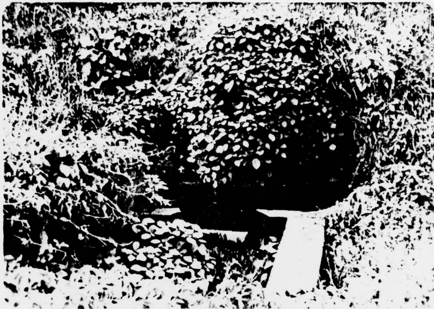
Photograph No. 11 Seepage weir on left abutment.
