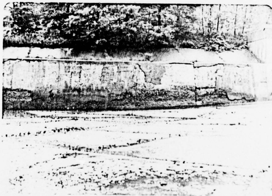
Photograph No. 10 Spalling in spillway discharge channel.
