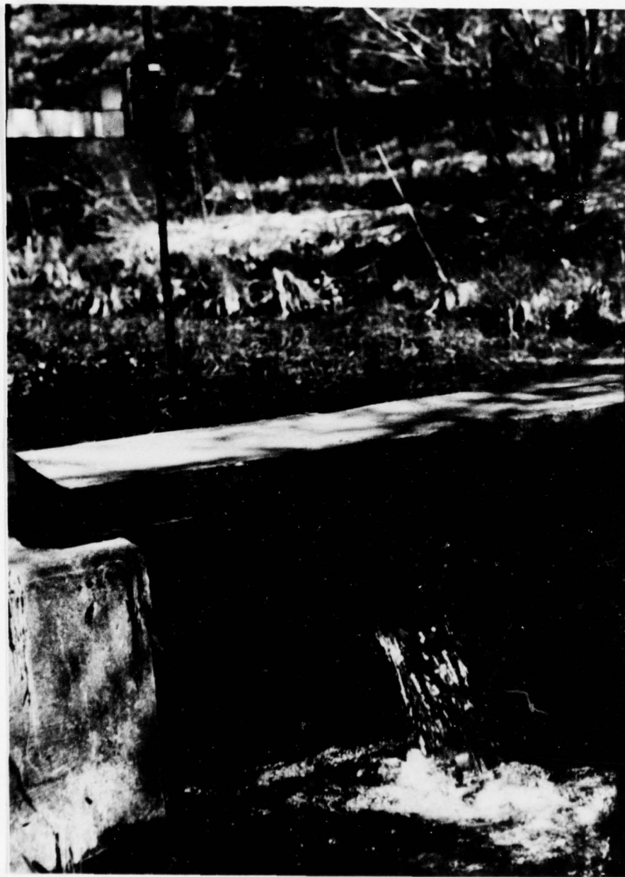
VIEW OF "V" NOTCH WEIR LOCATED DOWNSTREAM OF DIVERSION TUNNEL OUTLET STRUCTURE.
