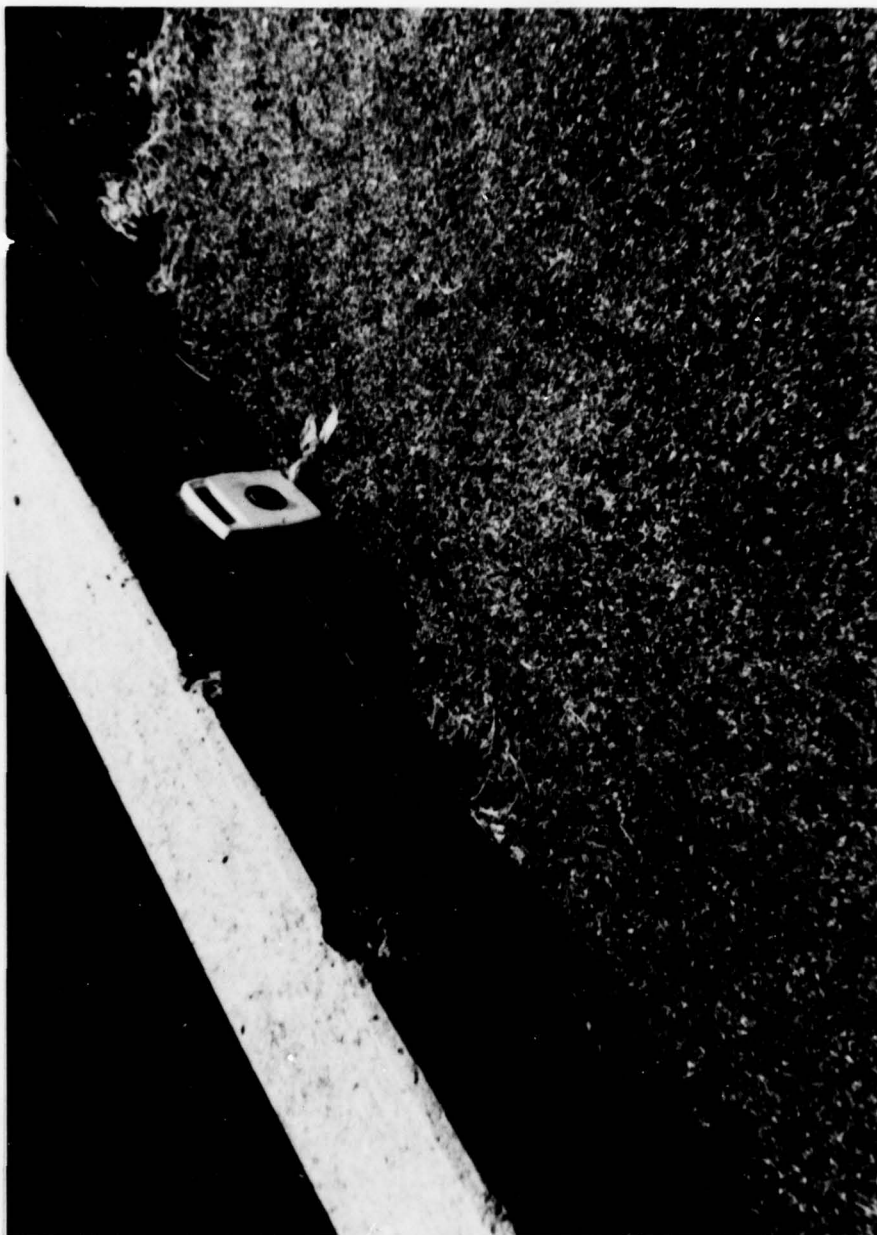
SETTLEMENT OF DAM CREST AT LEFT SPILLWAY WALL. PHOTO SHOWS 6 to 12 INCHES OF SETTLEMENT.
