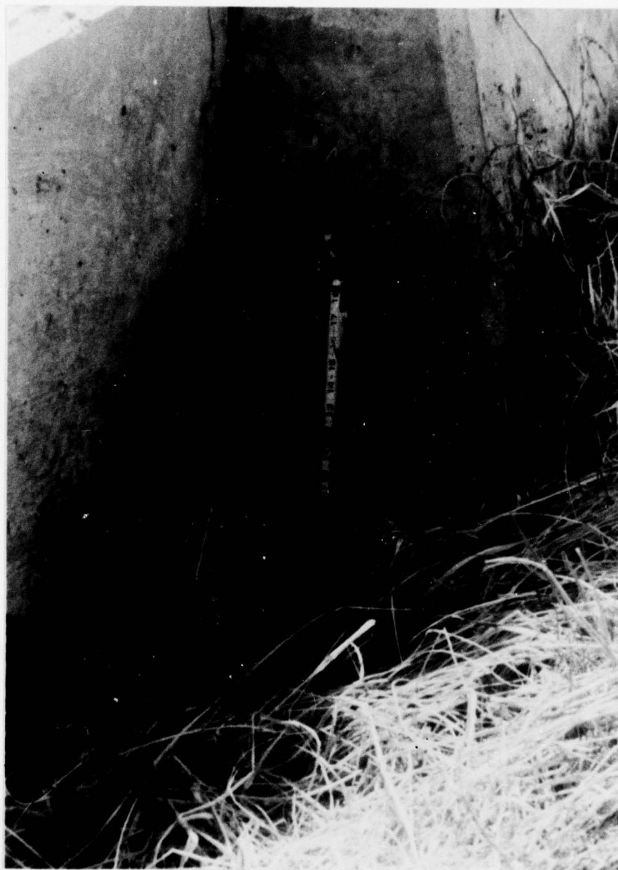
SETTLEMENT OF DOWNSTREAM SLOPE OF DAM AT LEFT SPILLWAY WALL. PHOTO SHOWS 12 INCHES OF SETTLEMENT.
