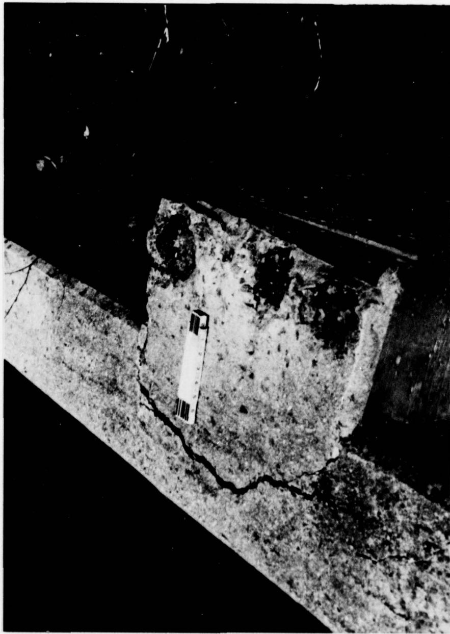
VIEW OF RETAINING WALL AND BUTTRESS SEPARATION ALONG RIGHT SIDE OF DISCHARGE CHANNEL.
