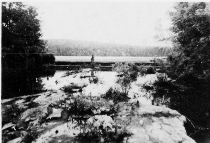
H. Spillway — Looking Upstream
