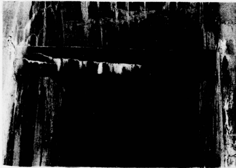
CONCRETE DETERIORATION OF UNDERFACE OF 45° INCLINED SLAB
