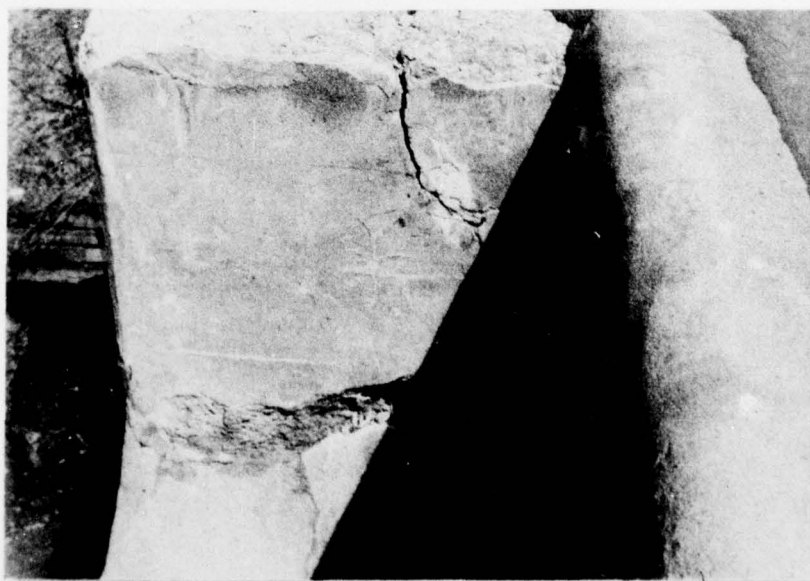
CLOSEUP VIEW SHOWING CONCRETE DETERIORATION AT NORTHERN END OF EMERGENCY SPILLWAY
