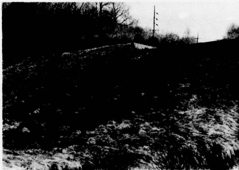
SLOUGH ON NORTHERN FACE OF EMBANKMENT
