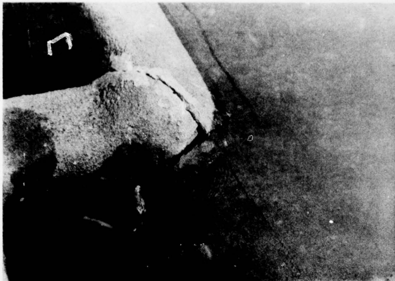
CLOSEUP VIEW OF LARGE CRACK AT NORTHERN END OF RECTANGULAR DROP-TYPE SPILLWAY
