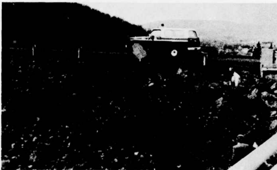
POOR GRADATION OF RIP RAP ON NORTH DAM EMBANKMENT
