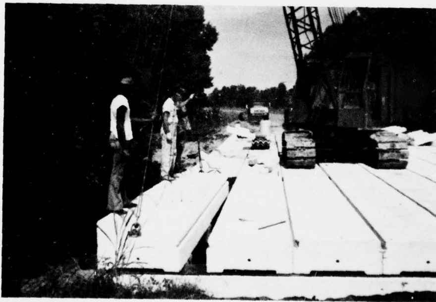
Photo D21. Positioning exterior channel girder
