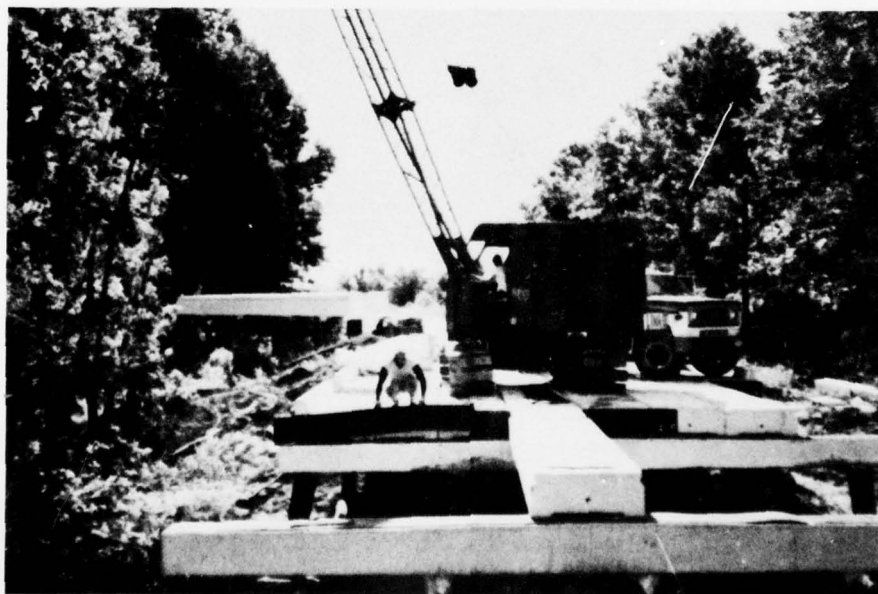
Photo D19. Positioning interior channel girders
