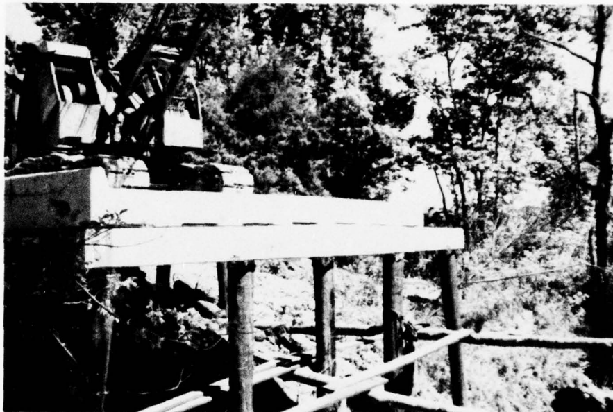
Photo D23. Upon completion of a bent, the crane is moved forward and the next bent is constructed using the same procedure
