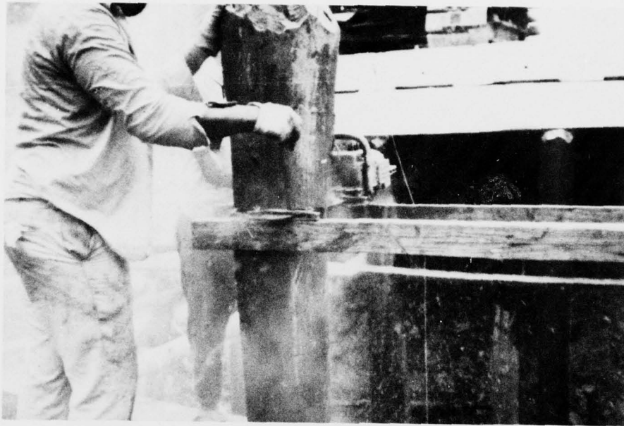
Photo D16. Cutting piles at desired elevation
