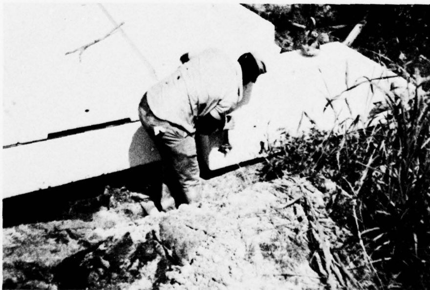
Photo D24. Installing precast abutment wing
