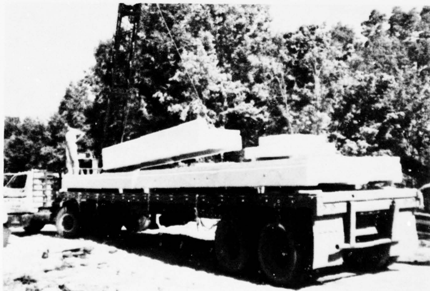
Photo D13. Typical transportation, precast plant to erection site
