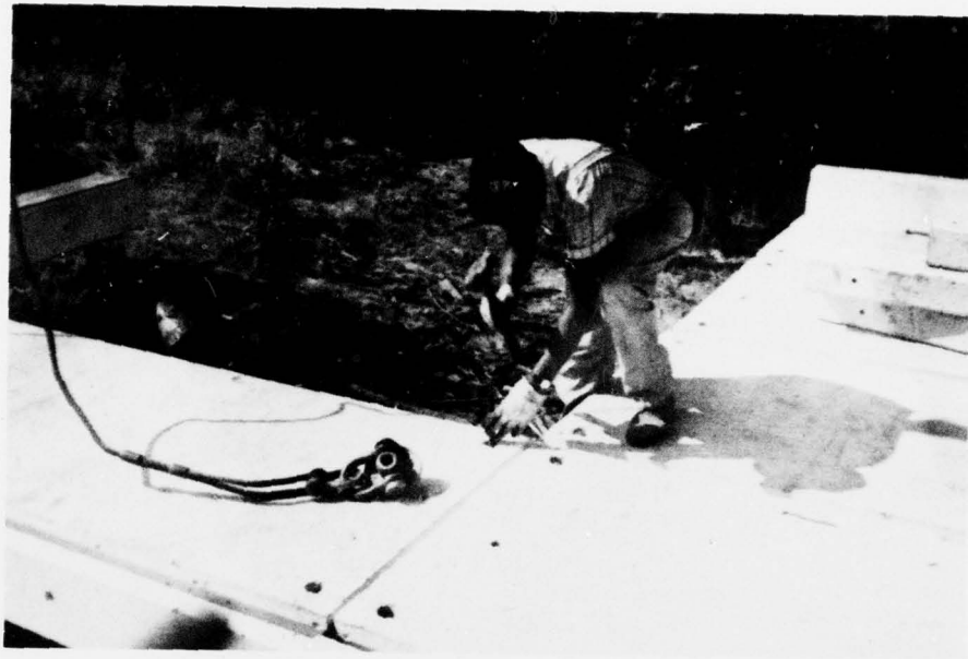
Photo D20. Inserting dowel pins through channel girder into pile cap
