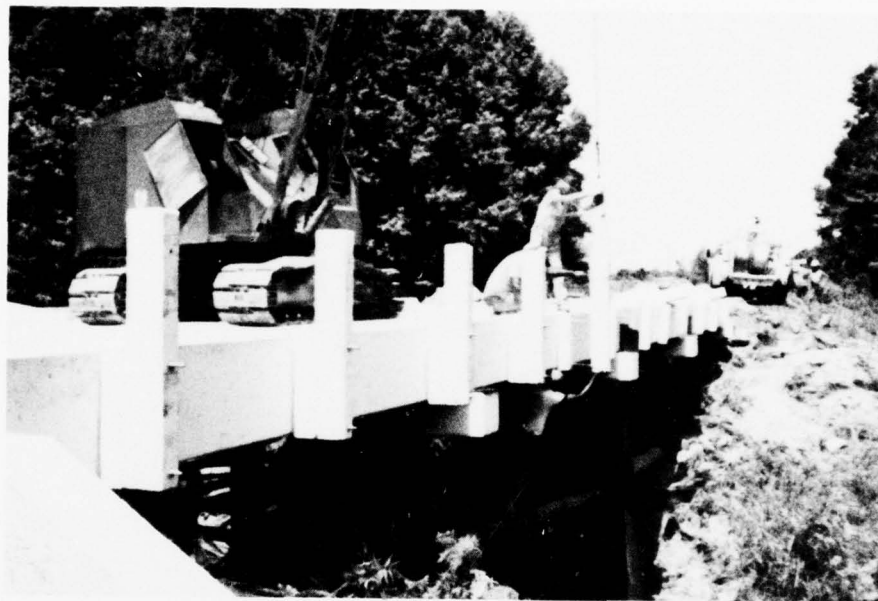
Photo D25. Installing precast guard rail posts
