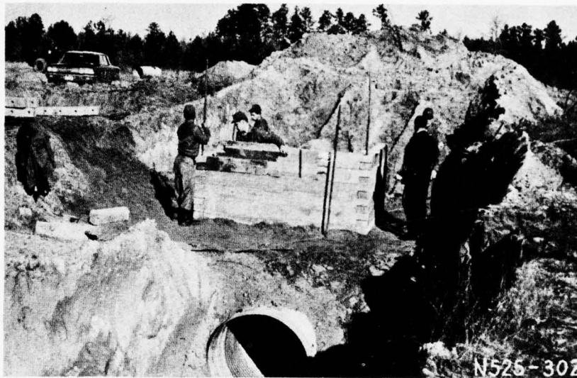
a. Installation of bunker (rear view)
