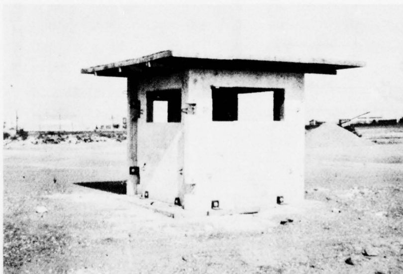
Figure 79. Precast concrete security bunker (from Reference 54)
