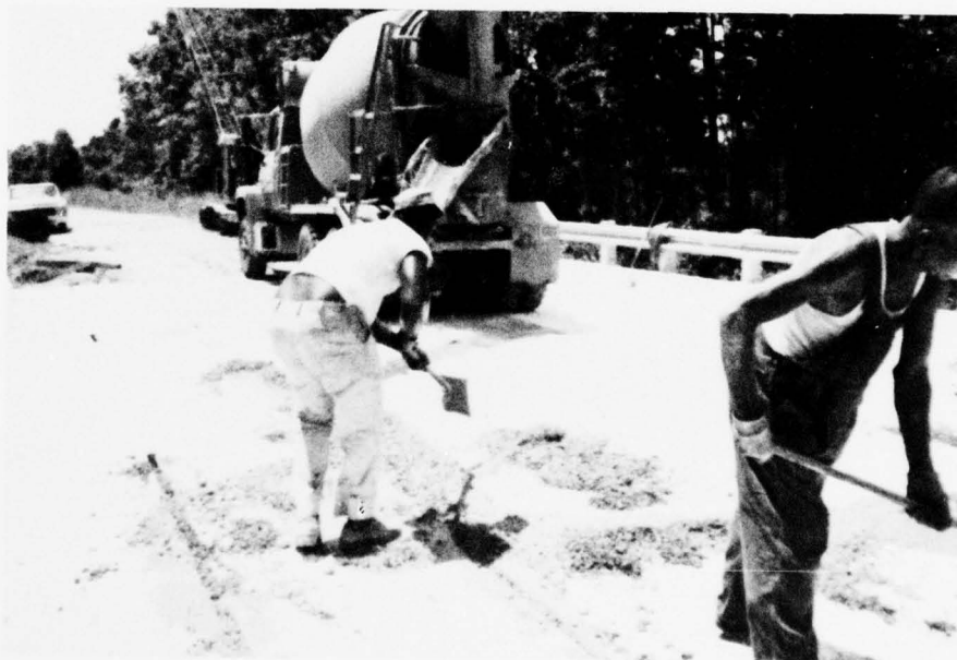
Photo D26. Concreting keyways and dowels
