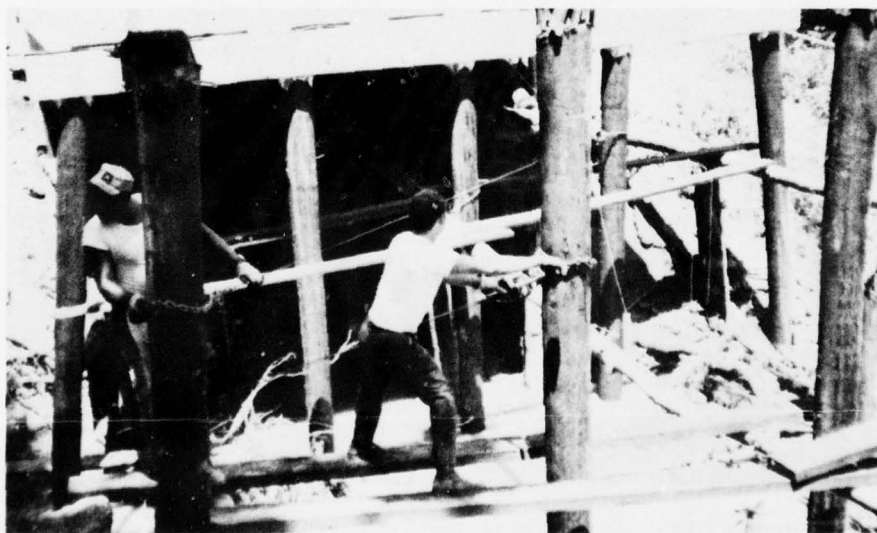
Photo D15. Using hand winches to obtain proper alignment of piles
