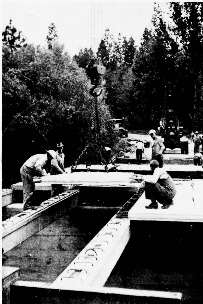
Figure 26. Erection of a bridge of precast beams and slabs (courtesy of Portland Cement Association)
