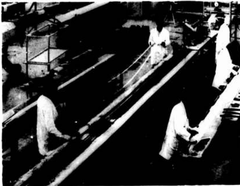
Fig. 23 Manufacture of the BO 105 Blade
