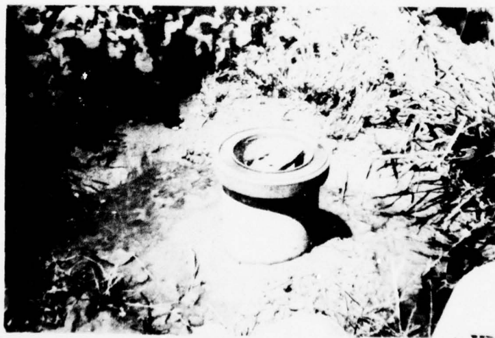
Alfalfa Valve Mounted on Concrete Pipe (not flowing)
