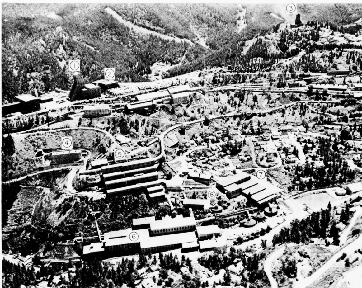
Homestake Gold Mine, Lead, South Dakota, is the Nation's Largest Operating Gold Mine Shafts and Hoists (1 & 3), Offices (2), Compressor (4), Mill (5), Cyanide Plants (6 & 7), Gold Refinery (8).
