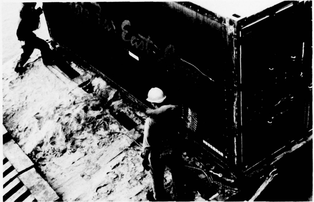
Figure 21. Tagline handlers placing sling spreader on container.
