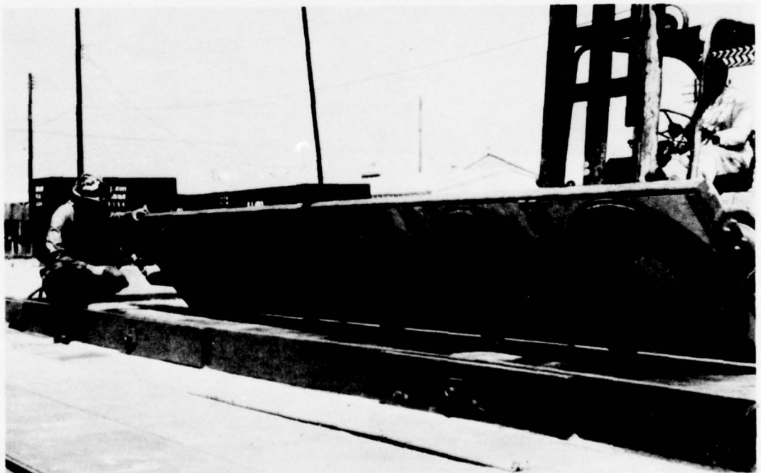
Figure 29. Air bearing transporter. Note air bearings used to support load.
