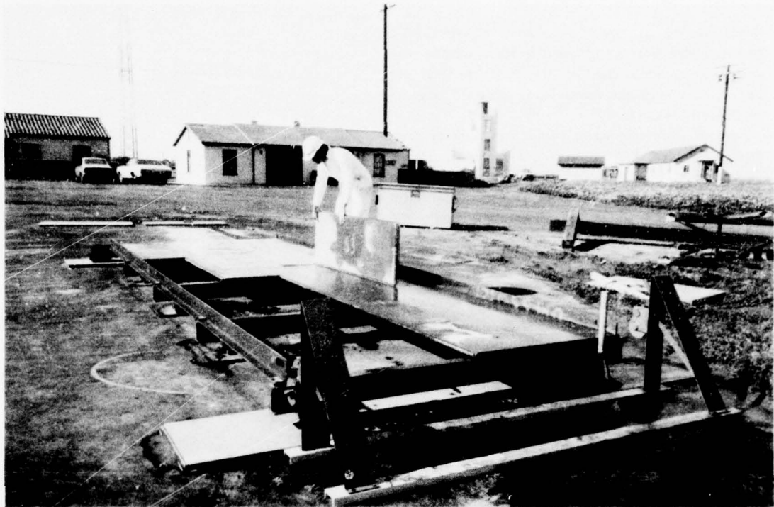
Figure 30. Partially assembled portable dock for air bearing system.
