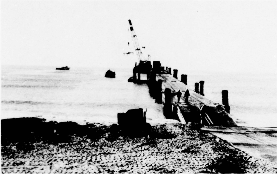
Figure 23. M8A1 steel matting roadway across beach to elevated causeway.
