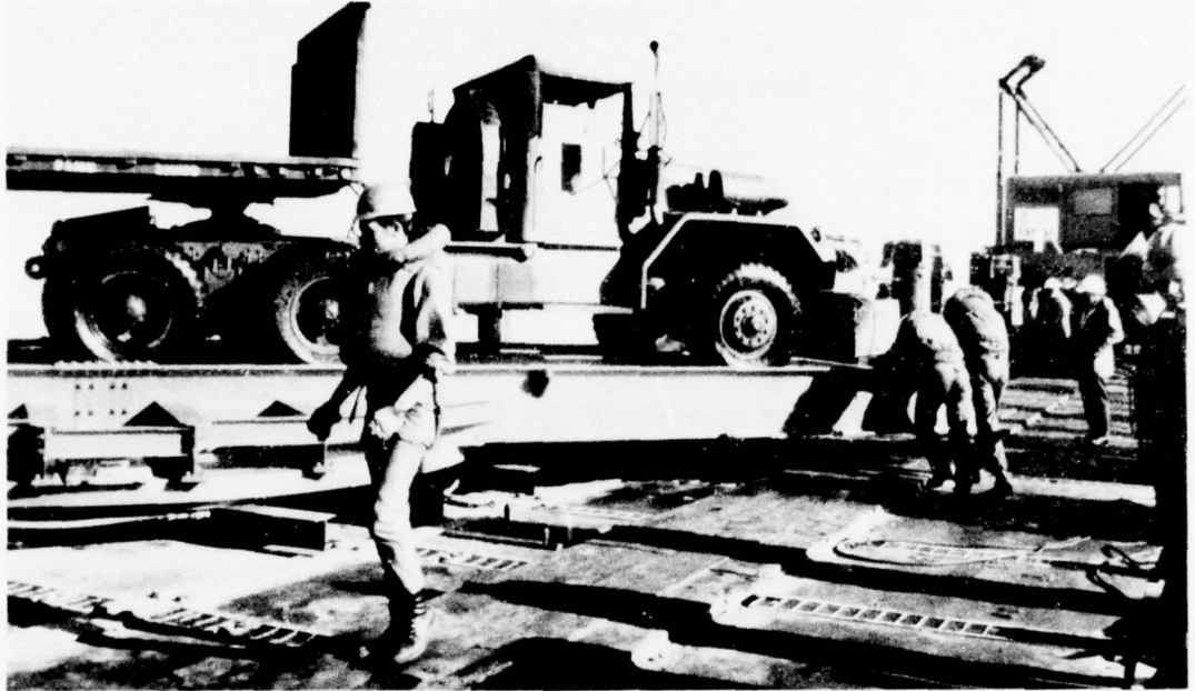
Figure 31. PHIBCB-ONE personnel turning truck/trailer 180 degrees on turntable.
