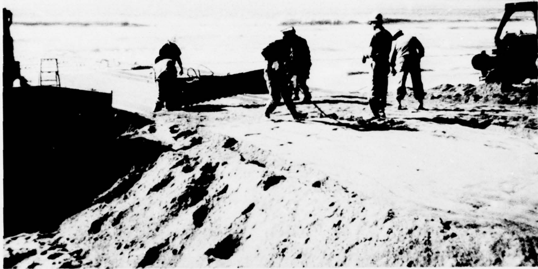
Figure 46. Beach transition ramp with built-up sand ramp.
