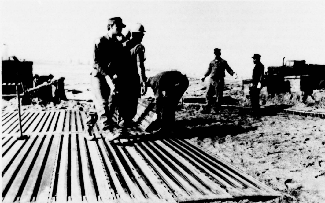
Figure 24. PHBCB-ONE crew installing M8A1 steel beach matting.
