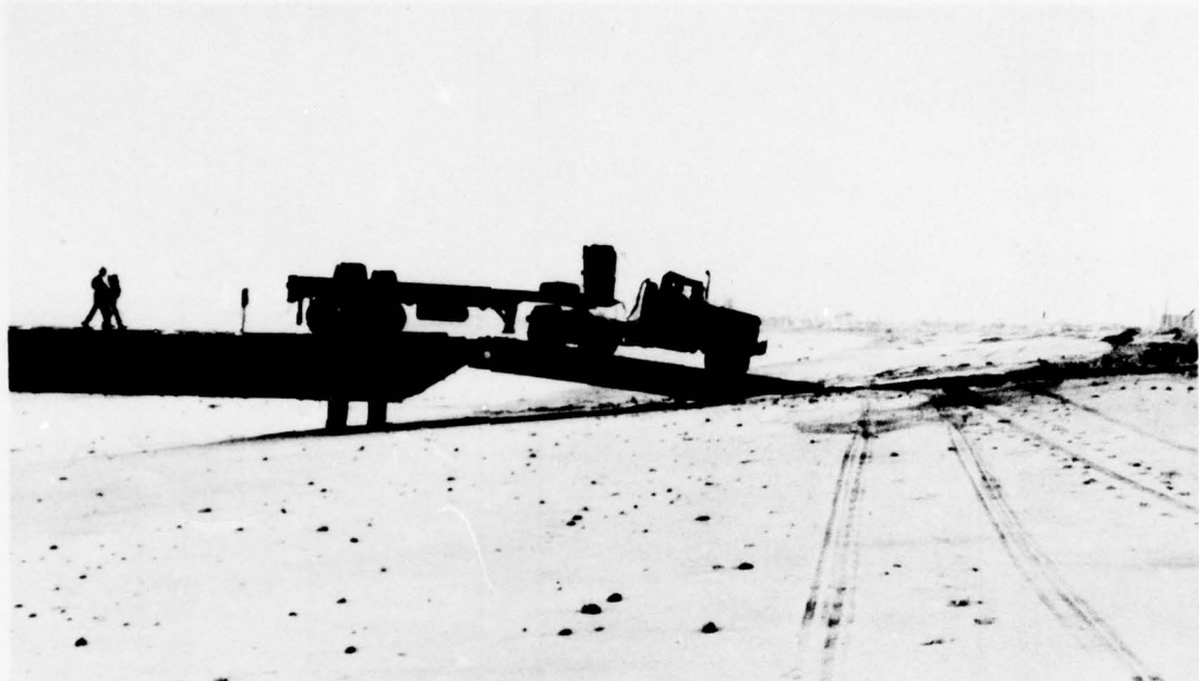
Figure 7. M52/M127 truck/trailer negotiating beach transition ramp from elevated causeway at low tide.
