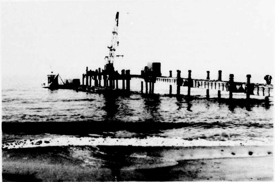
Figure 15. Causeway ferry alongside pierhead.
