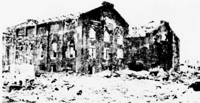
Figure 13a. Building 131A and B. Looking Northeast. Showing Destruction of Roofing. All Combustible Debris Burned. Note Burned-Over Area in Foreground From Which Fire Spread.
