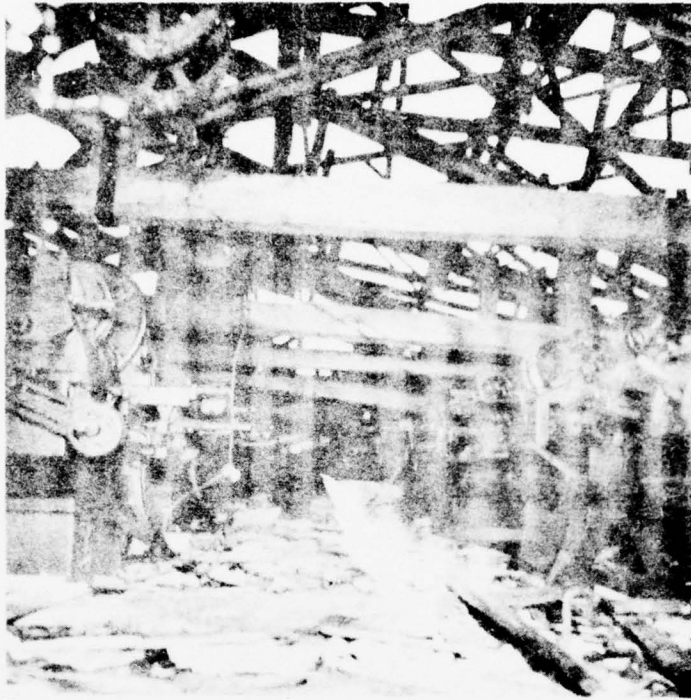
Figure 15. Building G, 6,000 Feet South of Gz, Looking West. A Wood-Frame, Light-Engineering Shop Collapsed as a Unit by Blast. No Fire.
