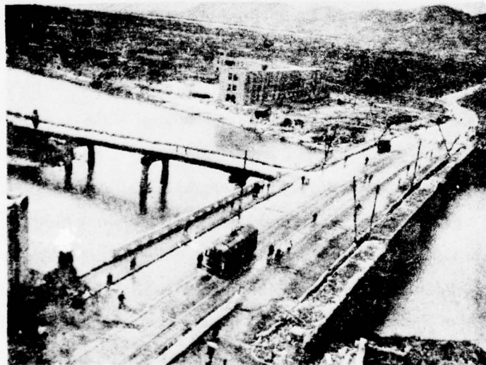
Figure 2. Intersection of Bridge 23 (Left) and Bridge 24 (Right). All Damage From Blast Effects. Bridge 23 (860 Feet to Gz, 2,170 Feet to Az). Bridge 24 (1,000 Feet to Gz, 2,230 Feet to Az).
