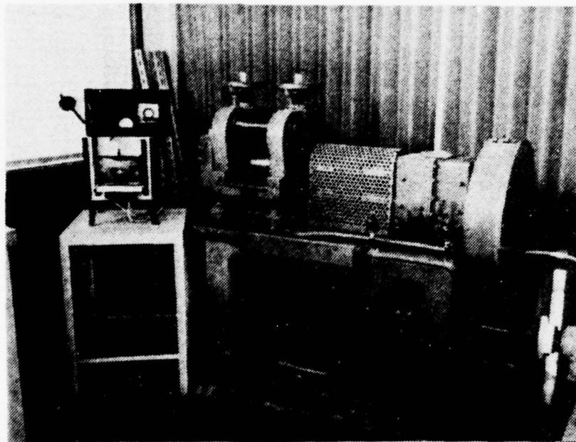
Figure 4 - WARMING FURNACE AND ROLLING MILL.
