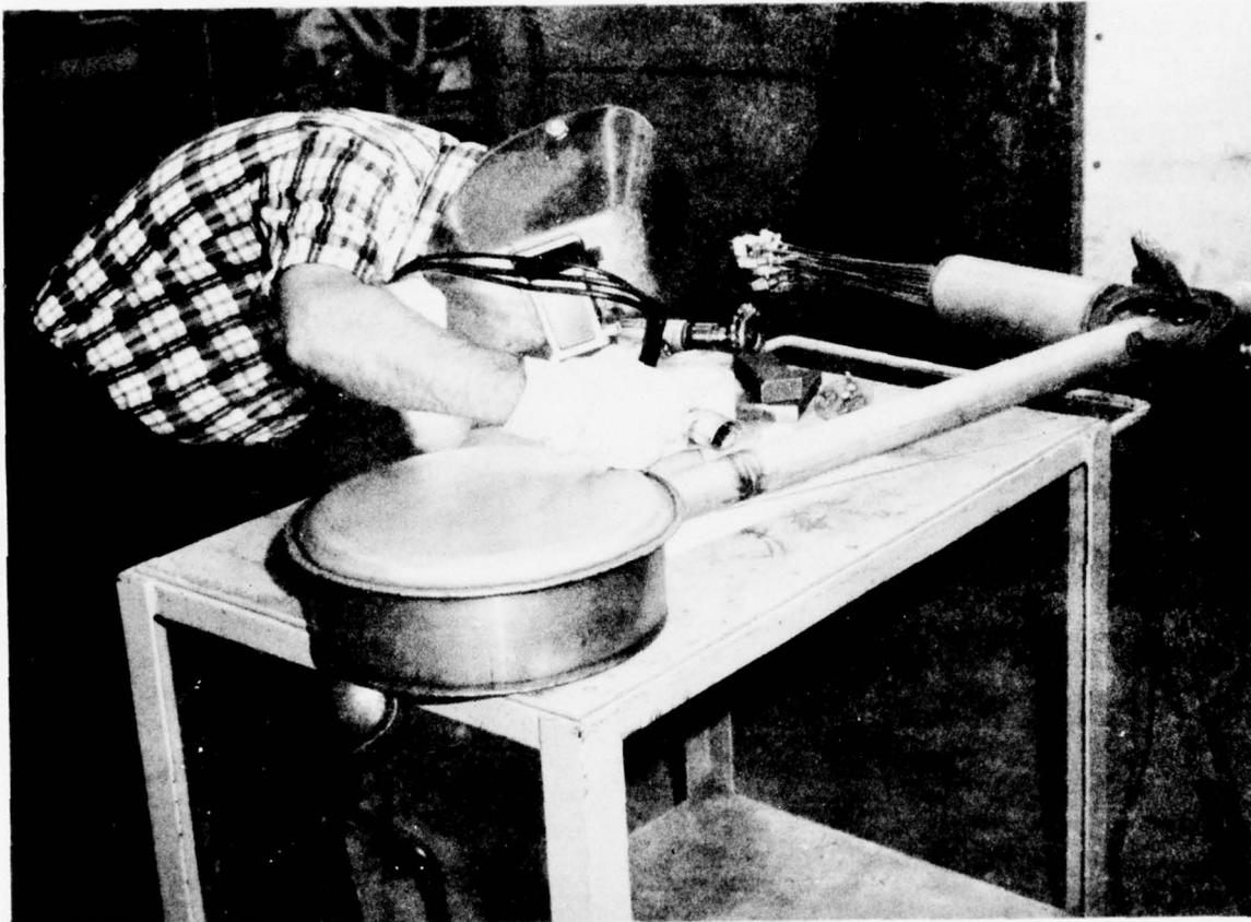
Figure 61. Laminated Wheel Blank Retort Being Welded After Backfilling with Argon.
