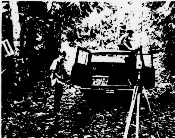
Fig. 5. Typical receiver setup. From left to right: HEMAC toroid coupled tree, PRC-74 set with whip, URM-85 field strength meter in vehicle, URM-85 whip on tripod, Gamboa Area, Panama Canal Zone, Sept. 1971.
