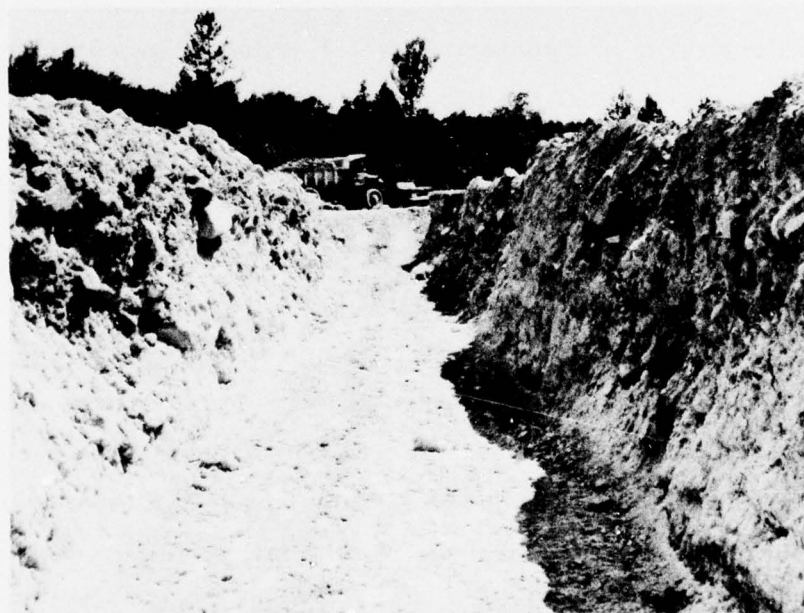
b. View south, inspection trench excavation
