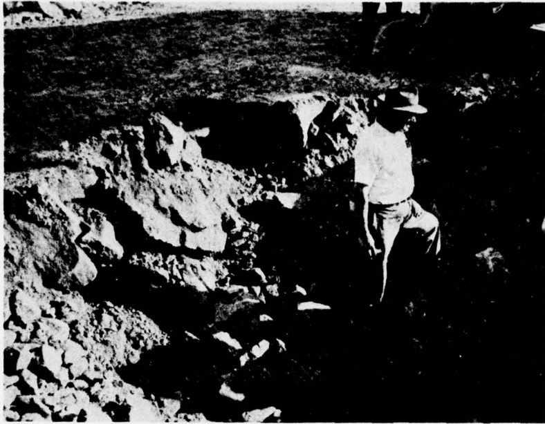
a. Second 3-ft lift
