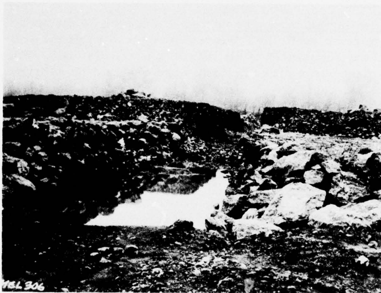
View of transverse cut through rock test fill embankments. From front to back:
