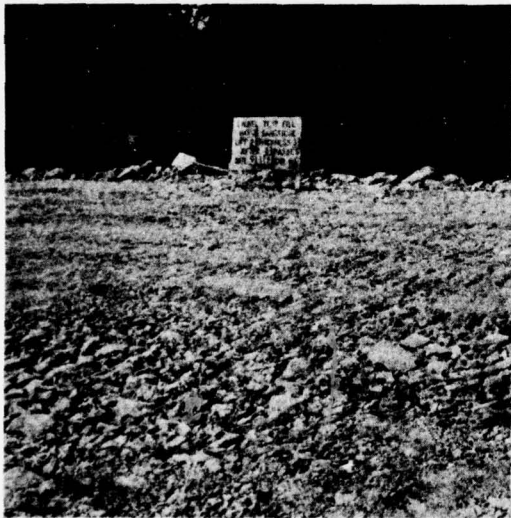
Second 3-ft lift (quarry run)
