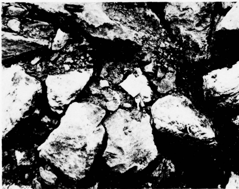
b. Closeup view of rock test fill 1 (6- to 18-in. weathered rock)
