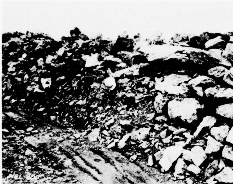
a. Section of rock test fill 4 (6- to 18-in. unweathered rock)
