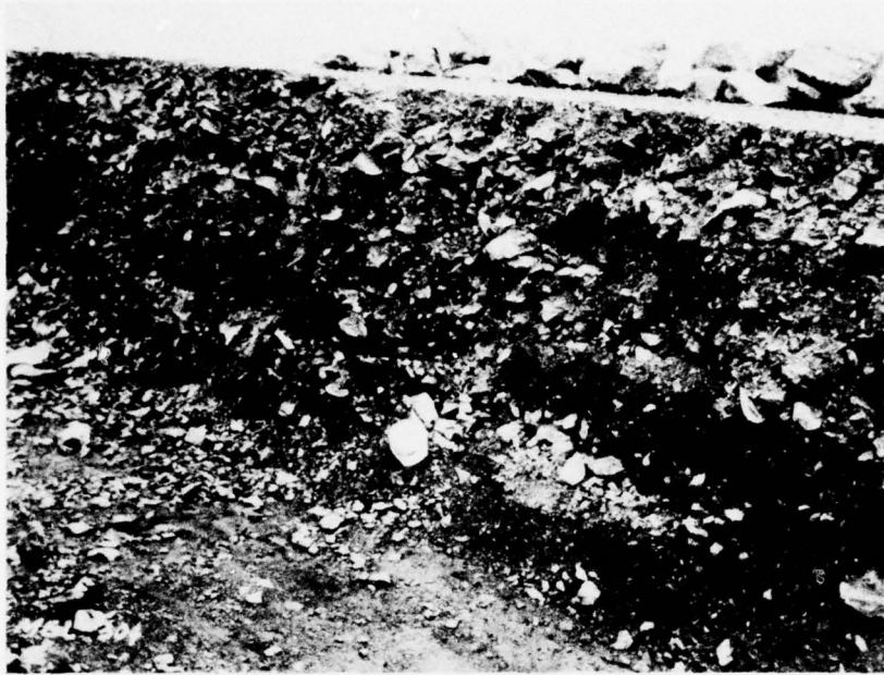
a. Section of rock test fill 2 (minus 6-in. weathered rock transition)
