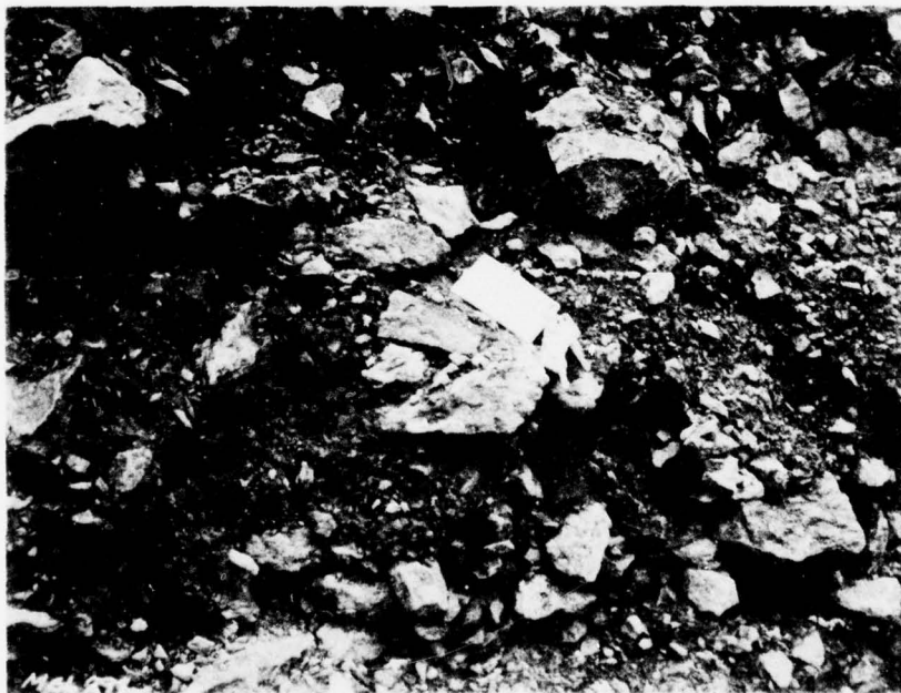
b. Closeup view of rock test fill 2 (minus 6-in. weathered rock transition)
