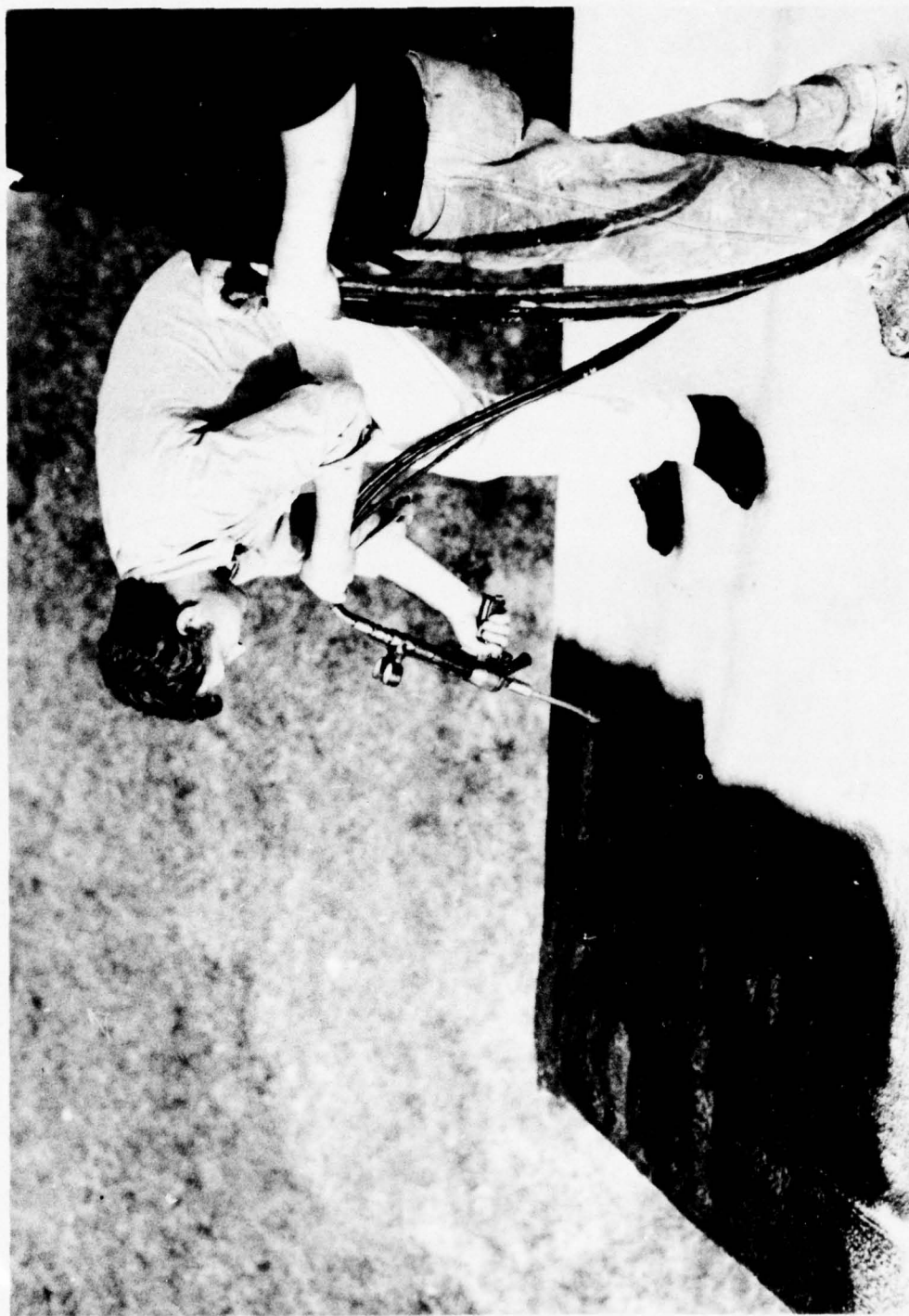
Figure 14. Spraying Black Butyl Base Coat of Catalyzed Butyl-Hypalon Coating (System 3) With Special Spray Gun
