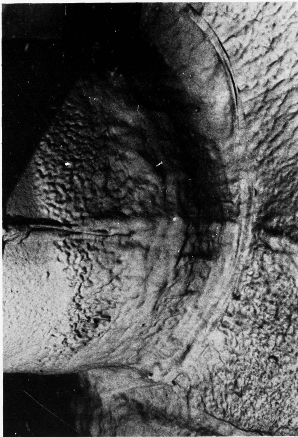
Figure 42. Fabric-reinforced Vent Flashing in System 2 Section, Performing Well After 18 Months of Weathering
