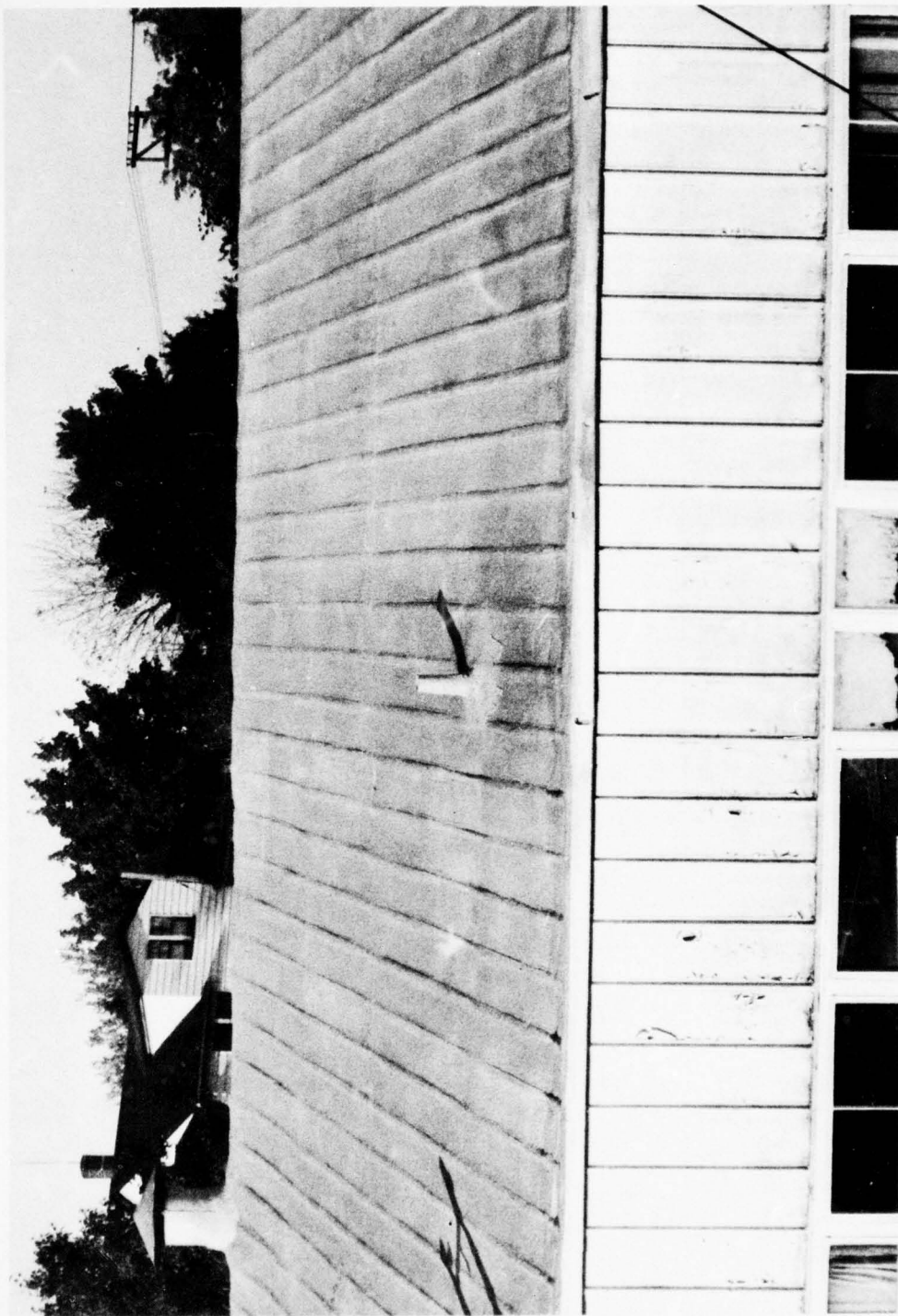
Figure 12. Completed South Side of Catalyzed Silicone Rubber Coating Section (System 1)
