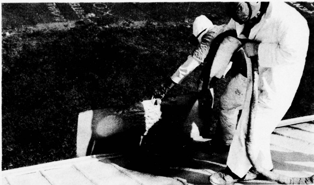
Figure 9. Spray-Application of Polyurethane Foam
