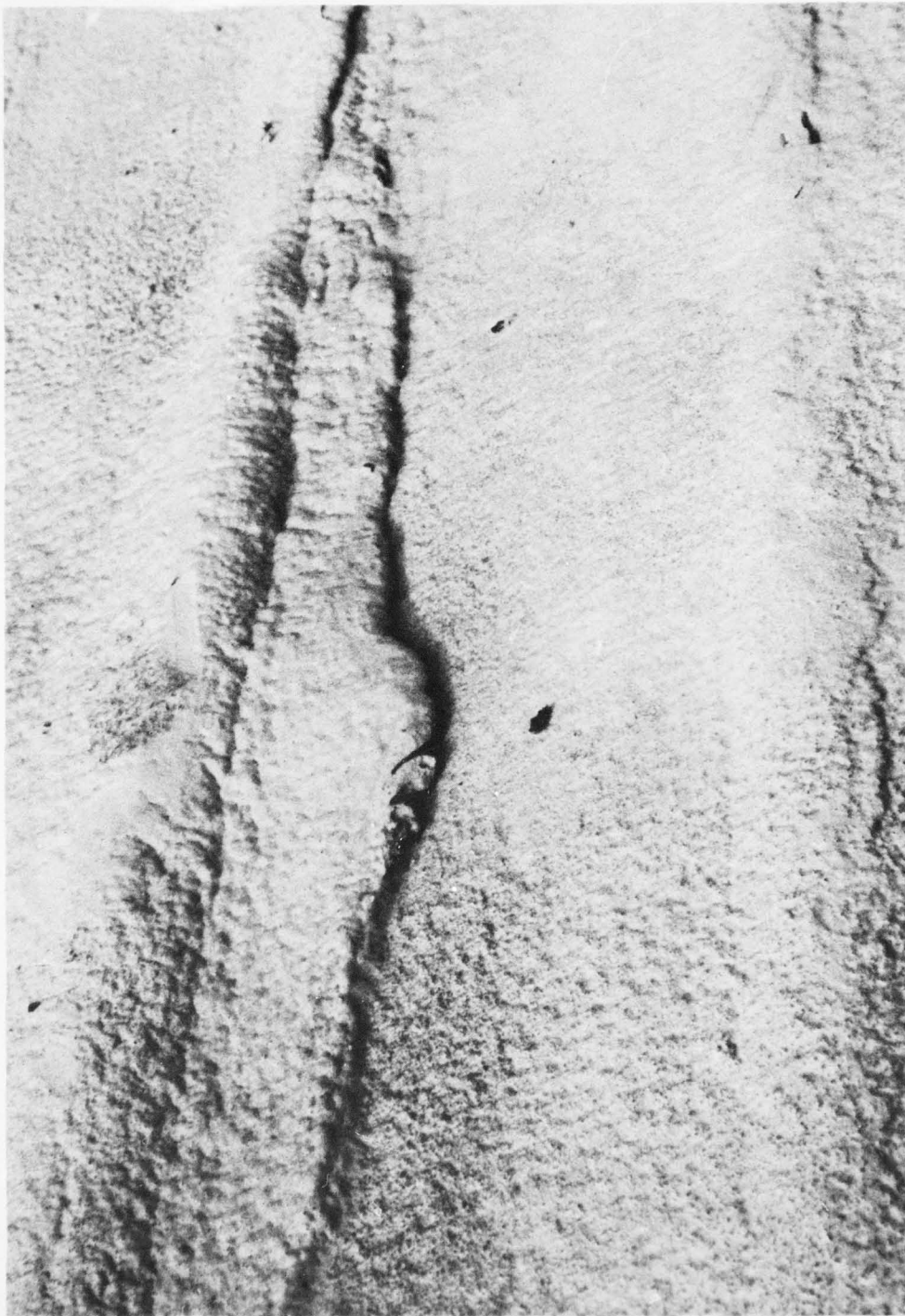
Figure 39. Poorly Constructed Overlap Joint Between System 3 Section and System 4 Section
