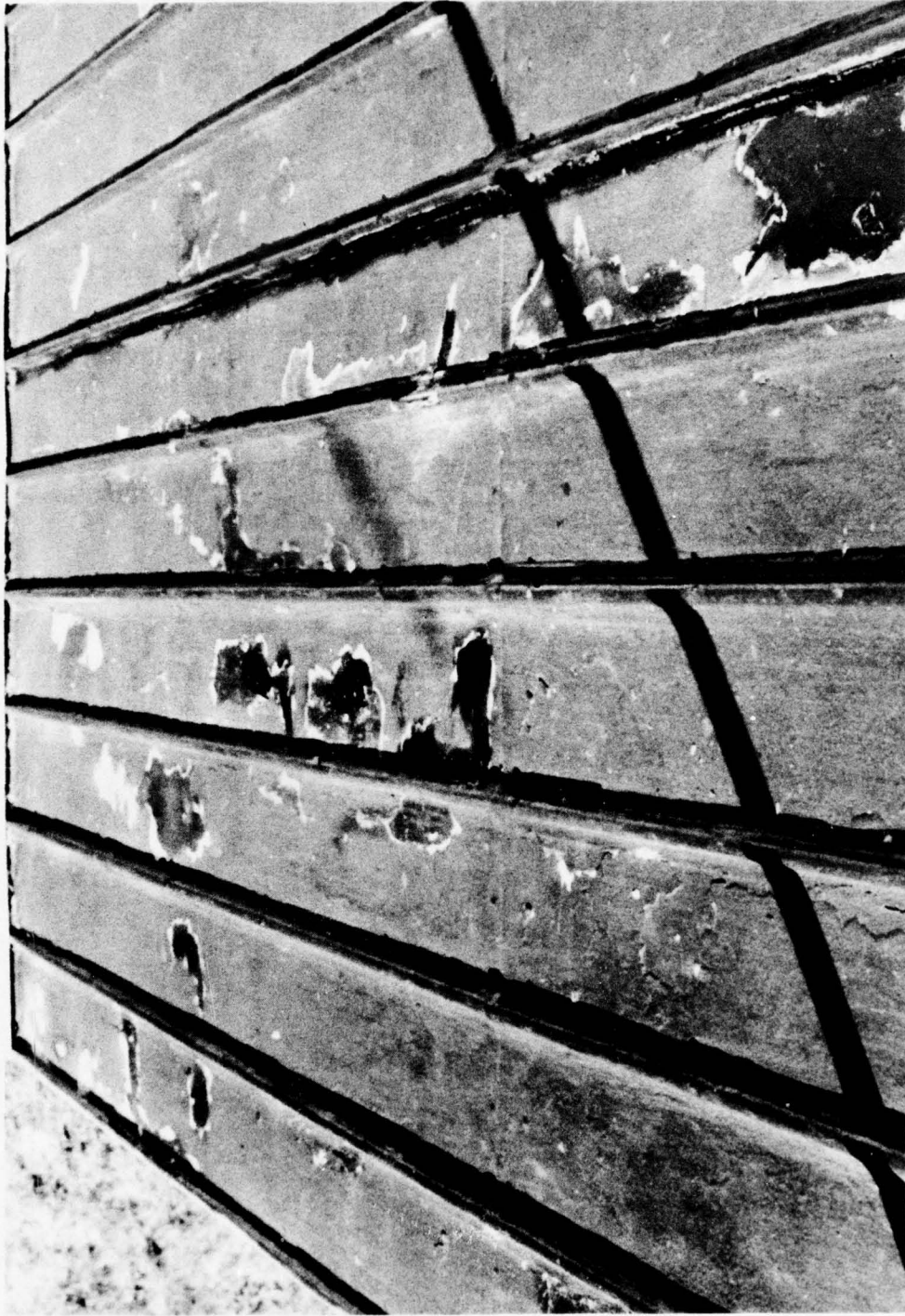
Figure 8. Spot-Primed Areas Ready For Foam Application
