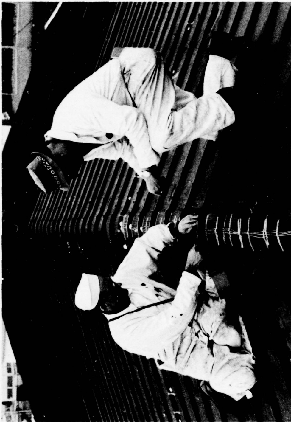
Figure 6. Installation of Thermocouple Wires
