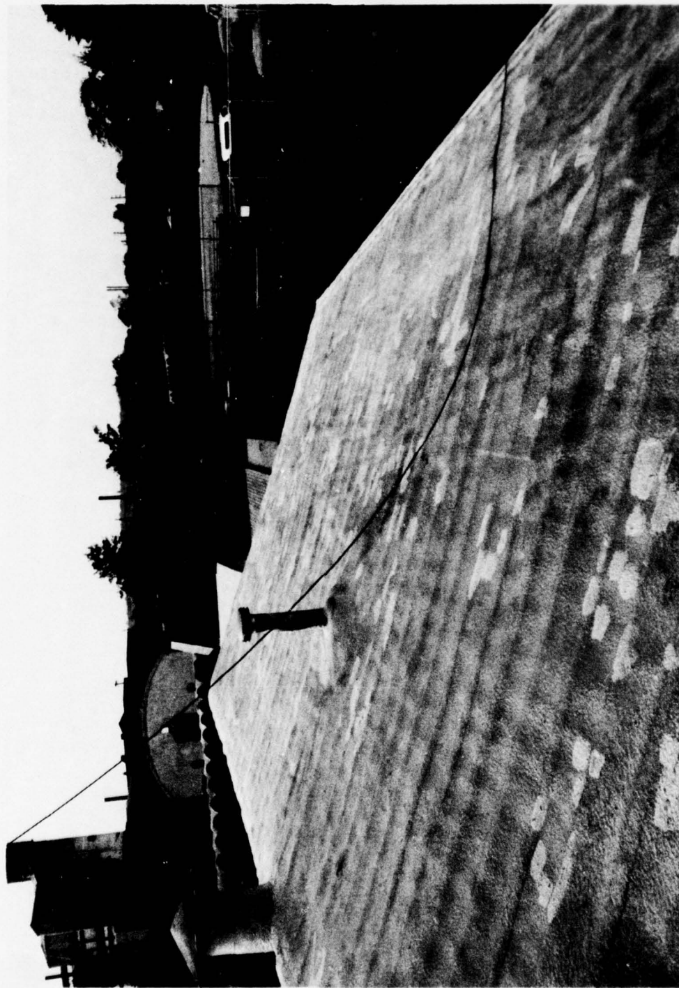
Figure 15. Completed North Side of Catalyzed Butyl-Hypalon Coating Section (System 3)
