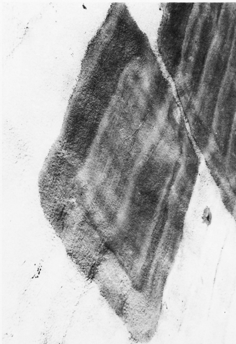
Figure 47. Repaired Areas Complete With Catalyzed Silicone Rubber Top Coat of System 1
