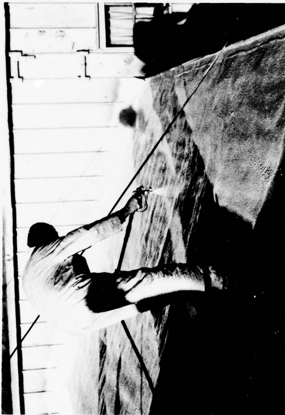
Figure 16. Spraying Hypalon Mastic Coating (System 4)
