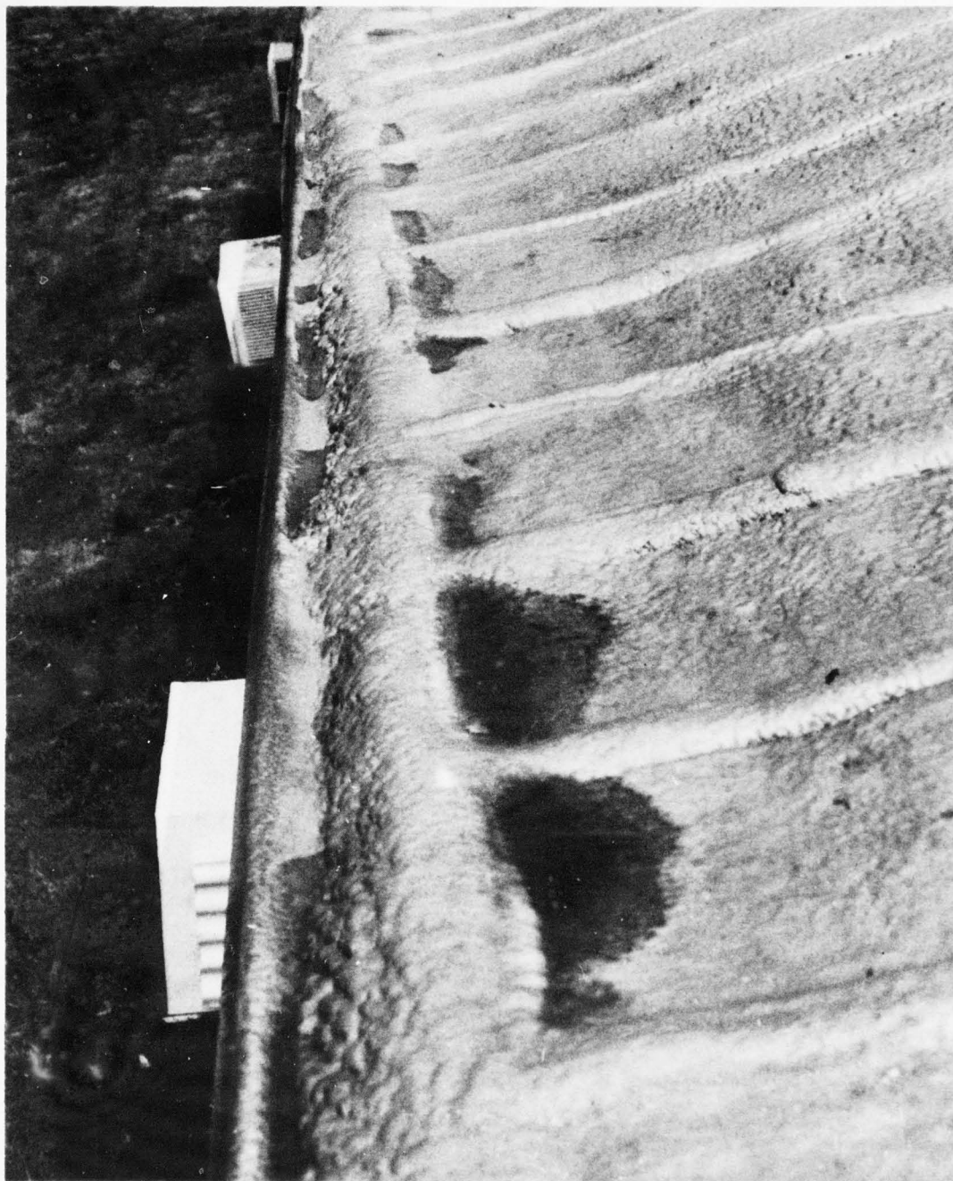
Figure 25. Ponded Water Along Gravel Stop in the System 1 Section
