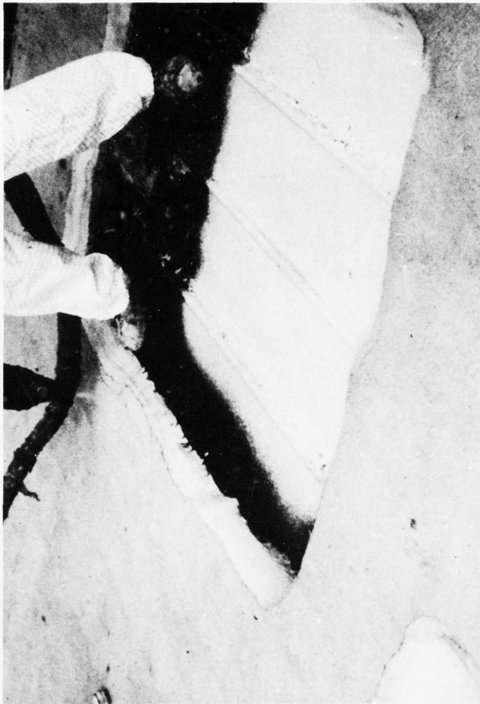
Figure 45. Application of New Foam in System 3 Section
