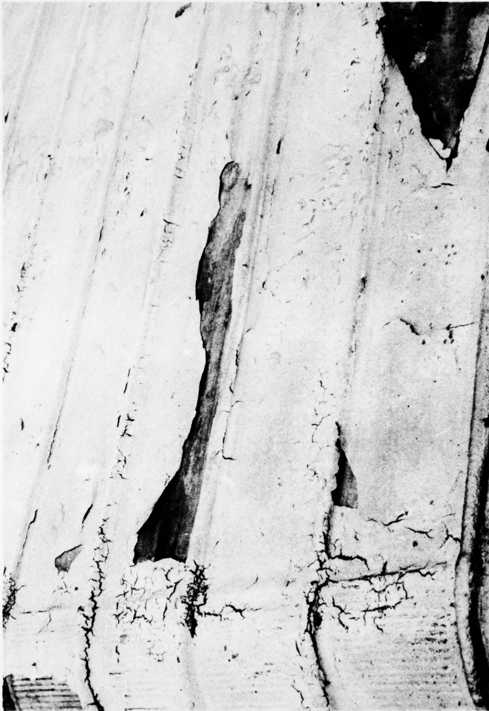
Figure 4. Roof Ridge Showing Cracked and Flaked Coatings, Before Reroofing
