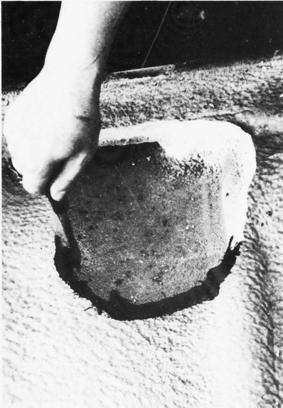
Figure 49. Repair of Large Bird-Pecked Area in System 2 Section
