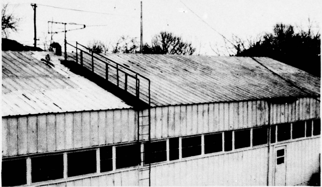
Figure 1. North Building Showing Accumulation of Old Coatings, Before Reroofing
