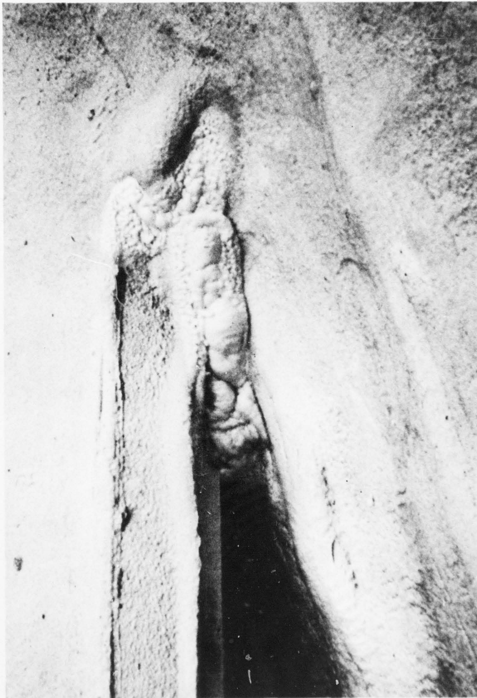
Figure 48. Junction of Boiler House Eave and South Building Filled With Foam
