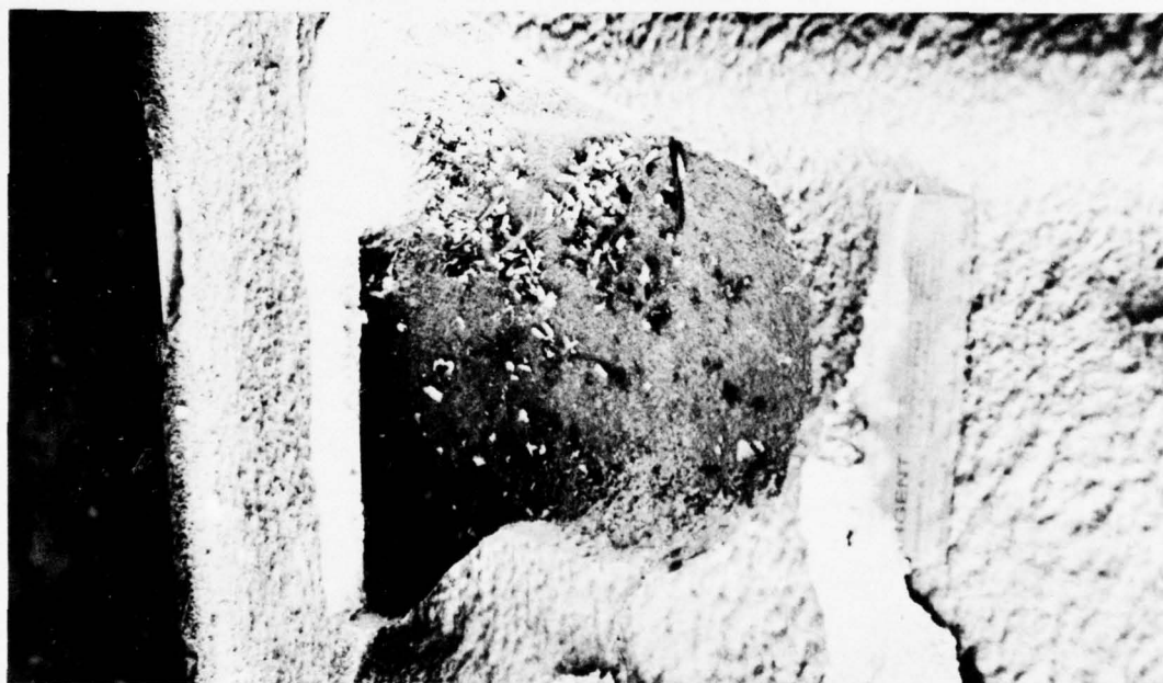
(b) Void Exposed When Coating Was Removed.
