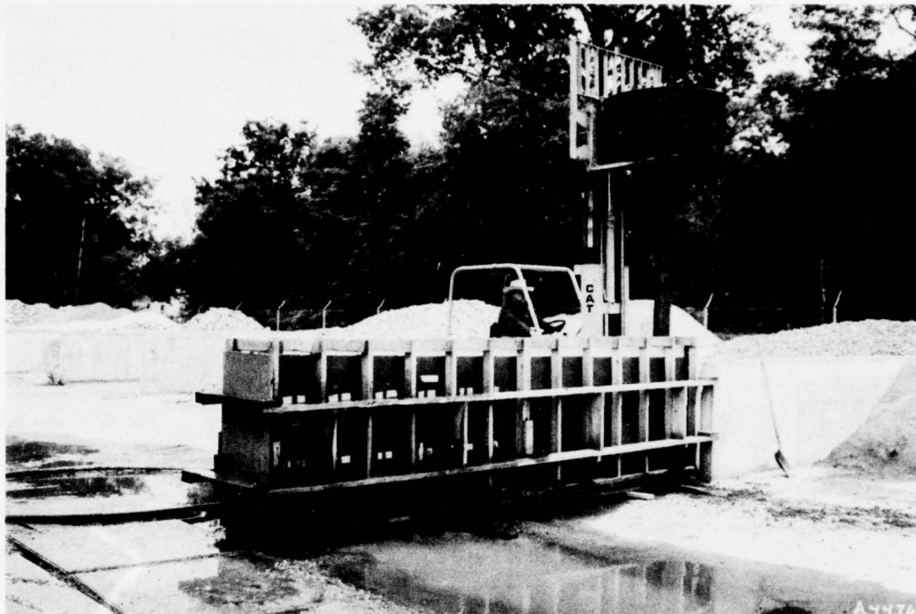
Figure 3. Form with the tremie pipe positioned at one end
